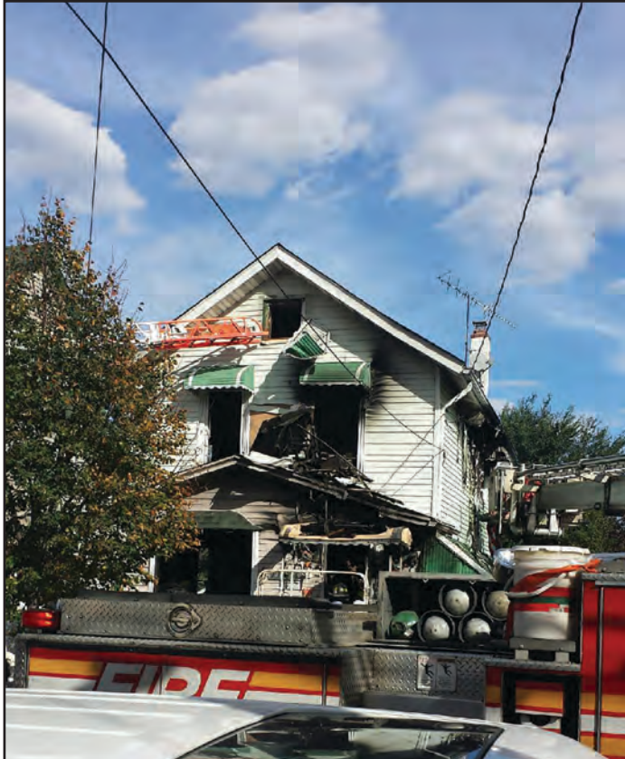
Aftermath of the fire that gutted a private dwelling on October 26, 2016, at Queens Box 75-8903.
