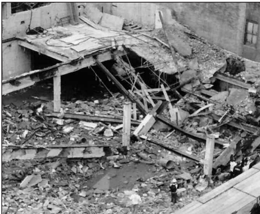
In order to reach the victim, FF Shepherd crawled into the void on his stomach, shoring the void as he moved in deeper. FF Shepherd initially used wood and other loose debris to quickly stabilize a one-ton piece of concrete that was hanging precariously above him. At any time, the concrete could have shifted, instantly crushing both rescuer and victim. The Manhattan building collapse scene from which FF Michael Shepherd removed a victim.
