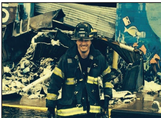
FM Robert J. Cox on the scene of an investigation; the March 12, 2014, gas explosion/collapse at Manhattan Box 55-1406. He is this year's recipient of the Deputy Commissioner Christine R. Godek Medal.
