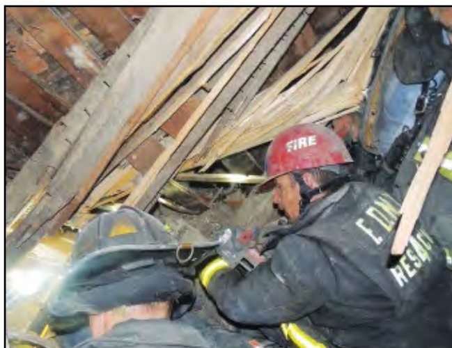
Rescue Firefighters take part in parallel extrication operations occurring on each side of the victim. Well into the operation, this area initially was covered by a partition and had to be reached by tunneling through the debris.
