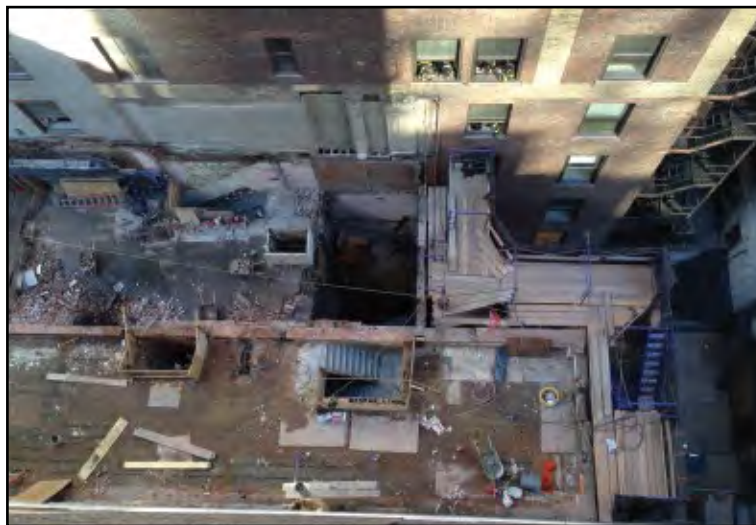
Aerial view of both buildings under demolition showing collapse in the rear section of the building.
