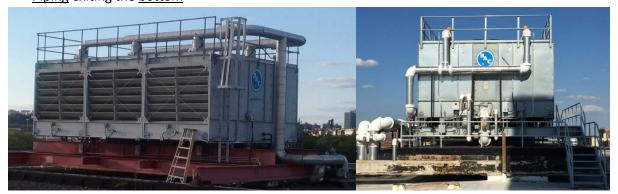
Some large cooling tower systems have more than one tower. Additionally, some cooling towers have more than one "cell" (sometimes called a "basin"). For example, an "eight-cell tower" is one cooling tower with eight cooling tower "cells." As long as the different cells inside a cooling tower and the
