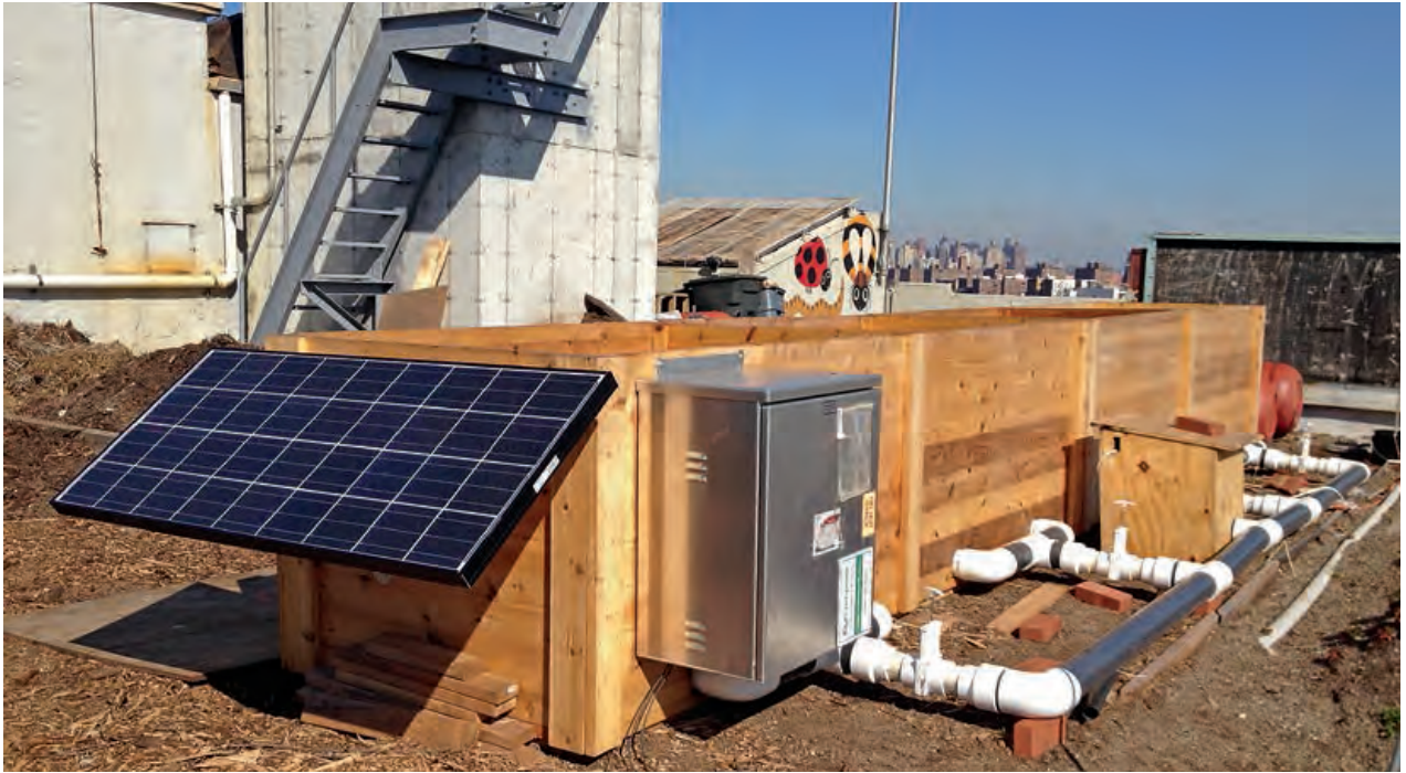
Solar powered forced aeration system in wood bins built by the NYC Compost Project hosted by Build It Green!NYC at Brooklyn Grange's rooftop farm in Long Island City.
