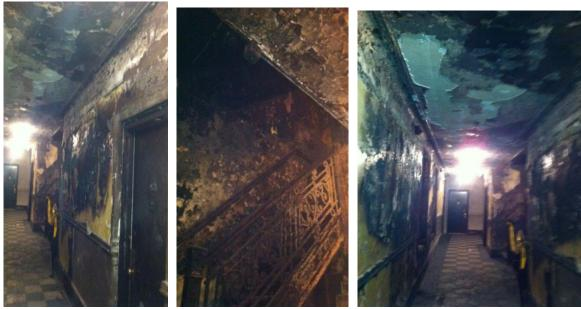
Pictures show the interior of the Bronx, NY shelter after the second mattress fire. There was severe smoke and fire damage in the hallways and stairwells.
