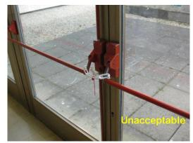
Picture shows a chained exit door, which is unacceptable.
