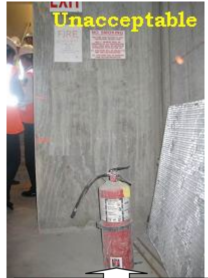
Improper floor placement of Fire Extinguisher.
