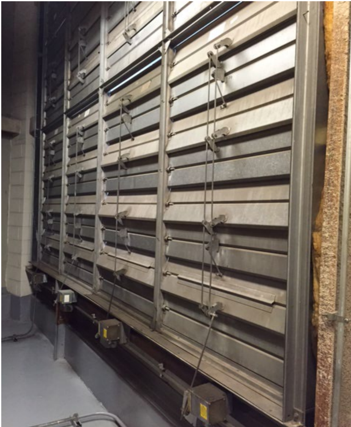
AIR LOUVER WITH ELECTRICAL MOTOR
