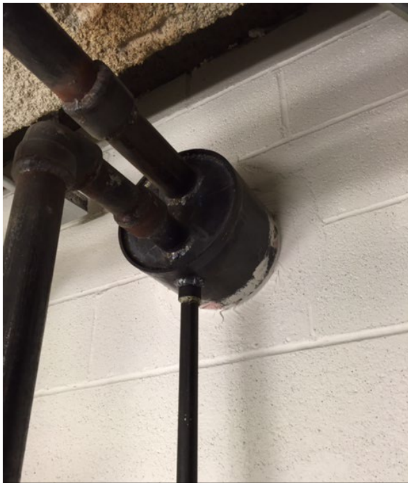
LEAK COLLECTOR INSIDE THE WALLS
