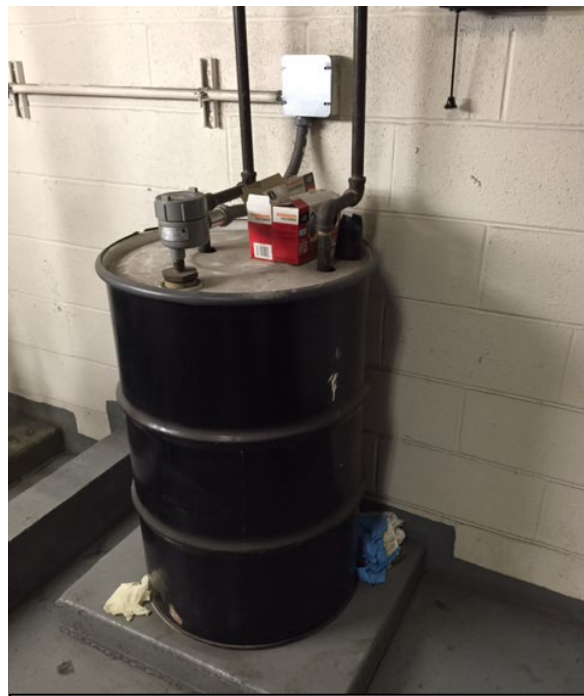
LEAK COLLECTOR WITH OIL LEVEL GAUGE
