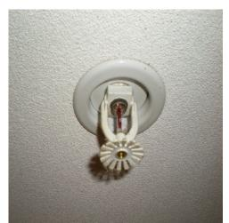
**Quick Response Ordinary Temperature Rated Factory Applied Finish Sprinkler**
