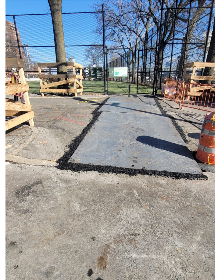
Steel plates over test pits on Jackson St. - February 2023
