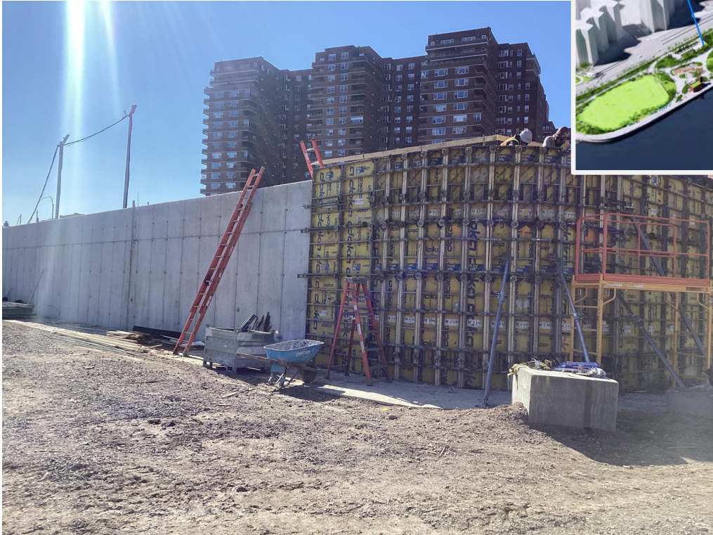
Maintenance and Operation Area #2 Retaining Wall - March 2023
