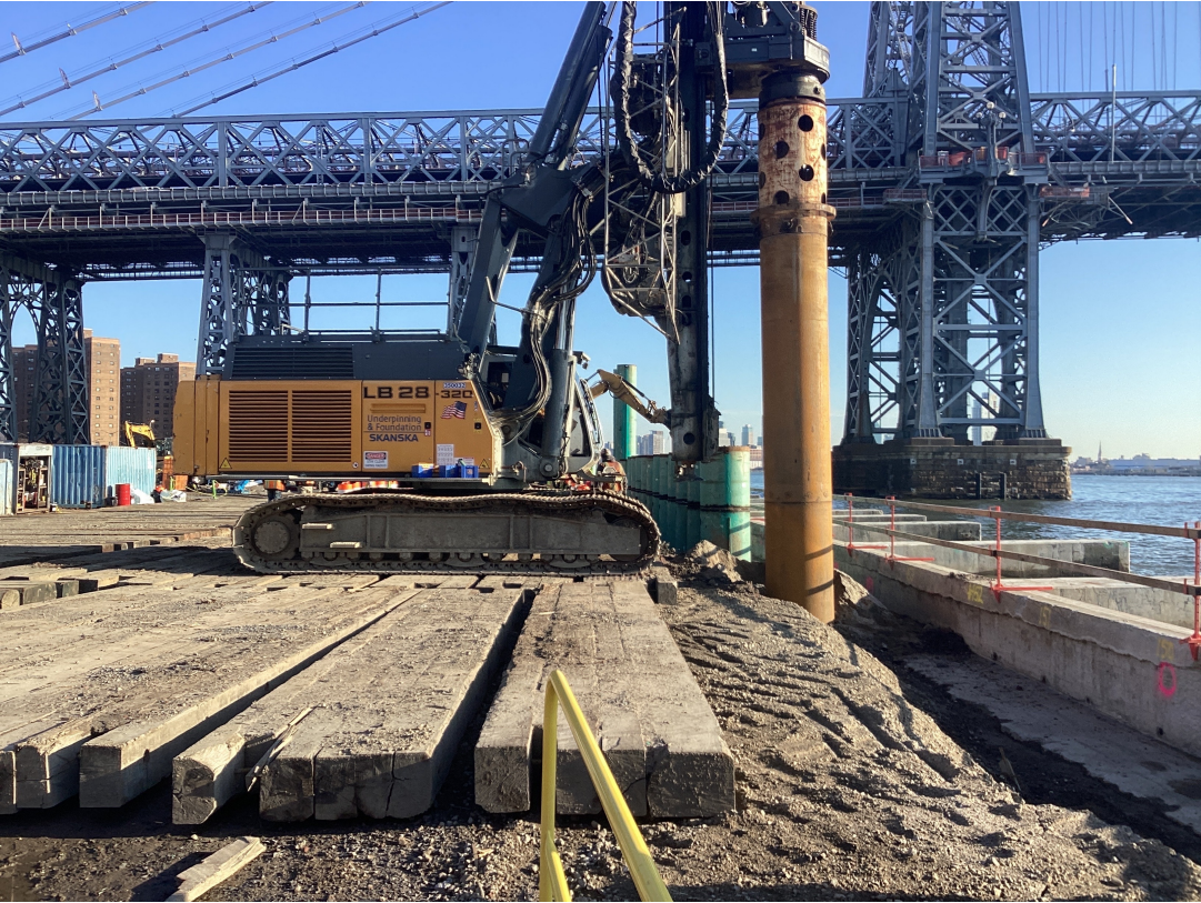
Combi-Wall Pre-Drilling and Installed Piles along Esplanade - March 2023
