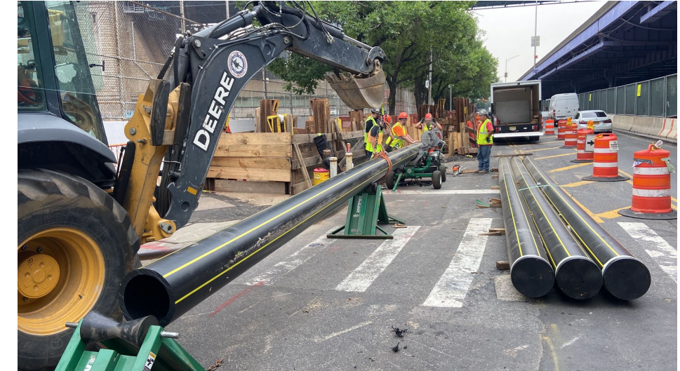
Gas main installation
