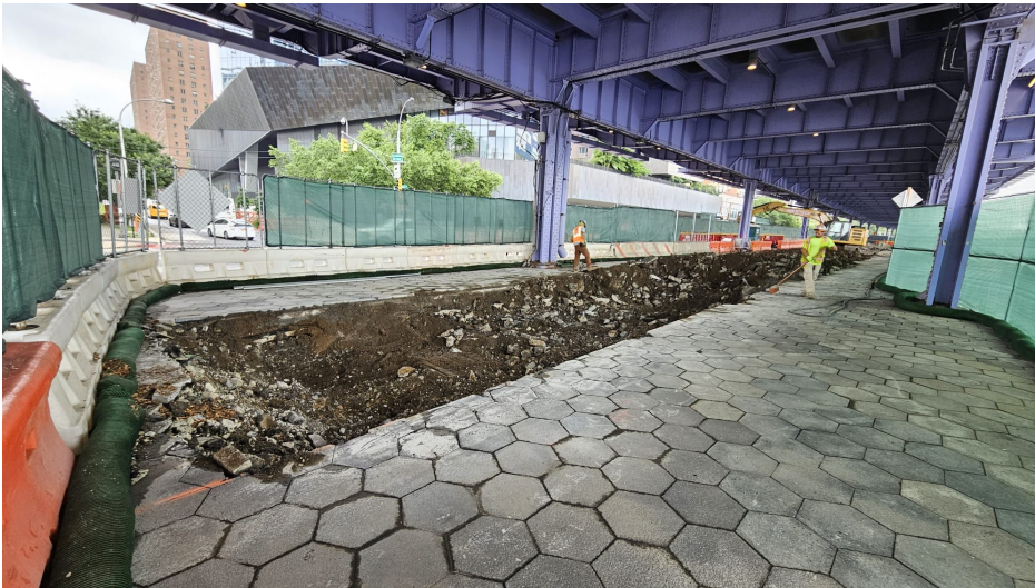
Excavation for floodgate foundation
