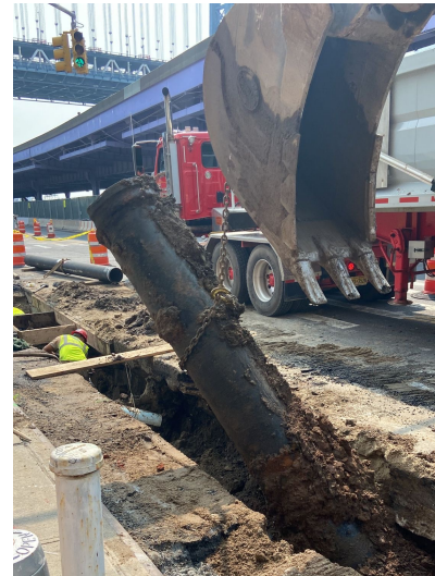
Water main removal
