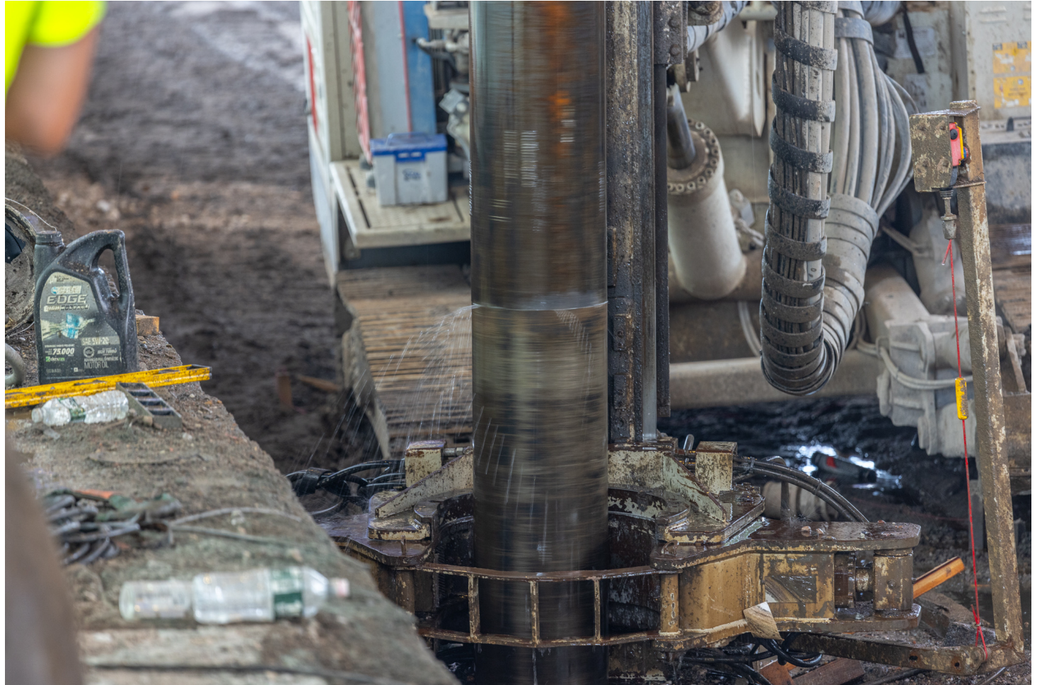
Micropile Installation – September 2023
