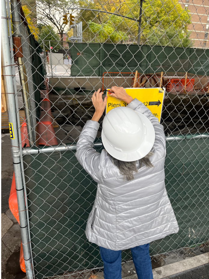
Installing temporary wayfinding signage October 2023
