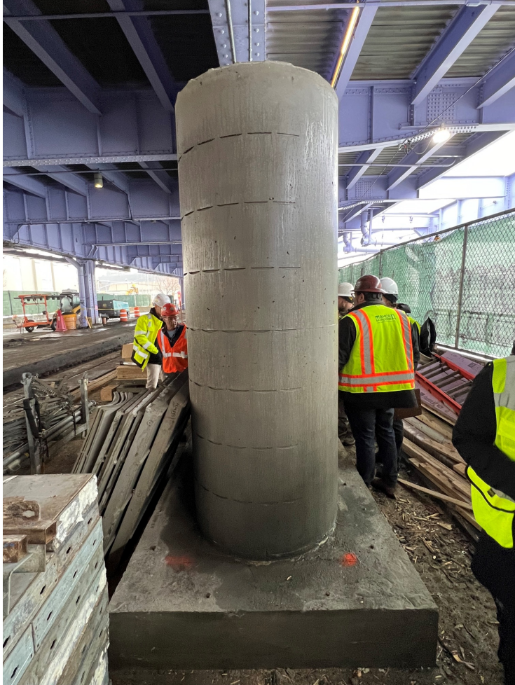
Floodwall mockup - February 2024
