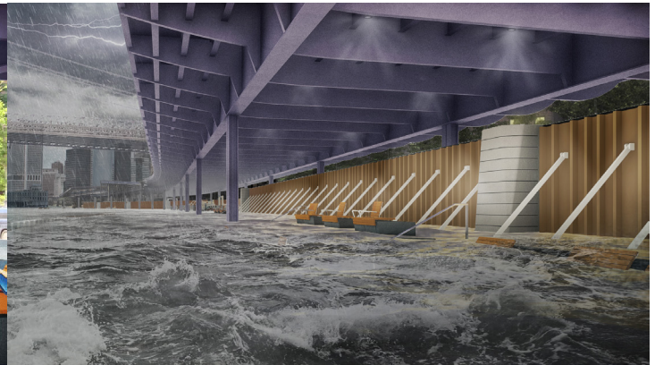
Activated Flip Up Gates at Catherine Slip During Storm
