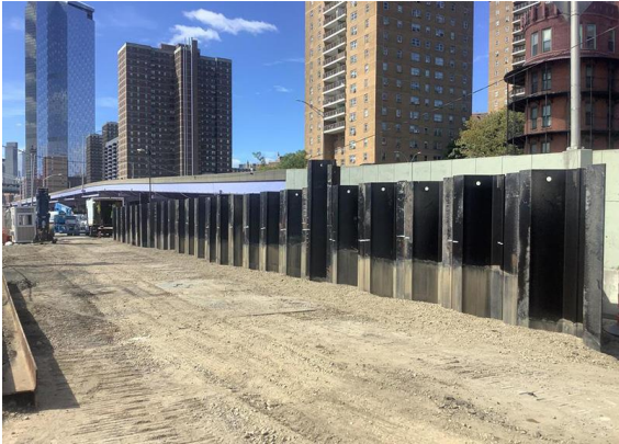
Sheet pile, Combi Wall, Sewer expansions
