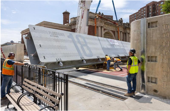
Floodgate, Asser Levy Playground, Flood wall
