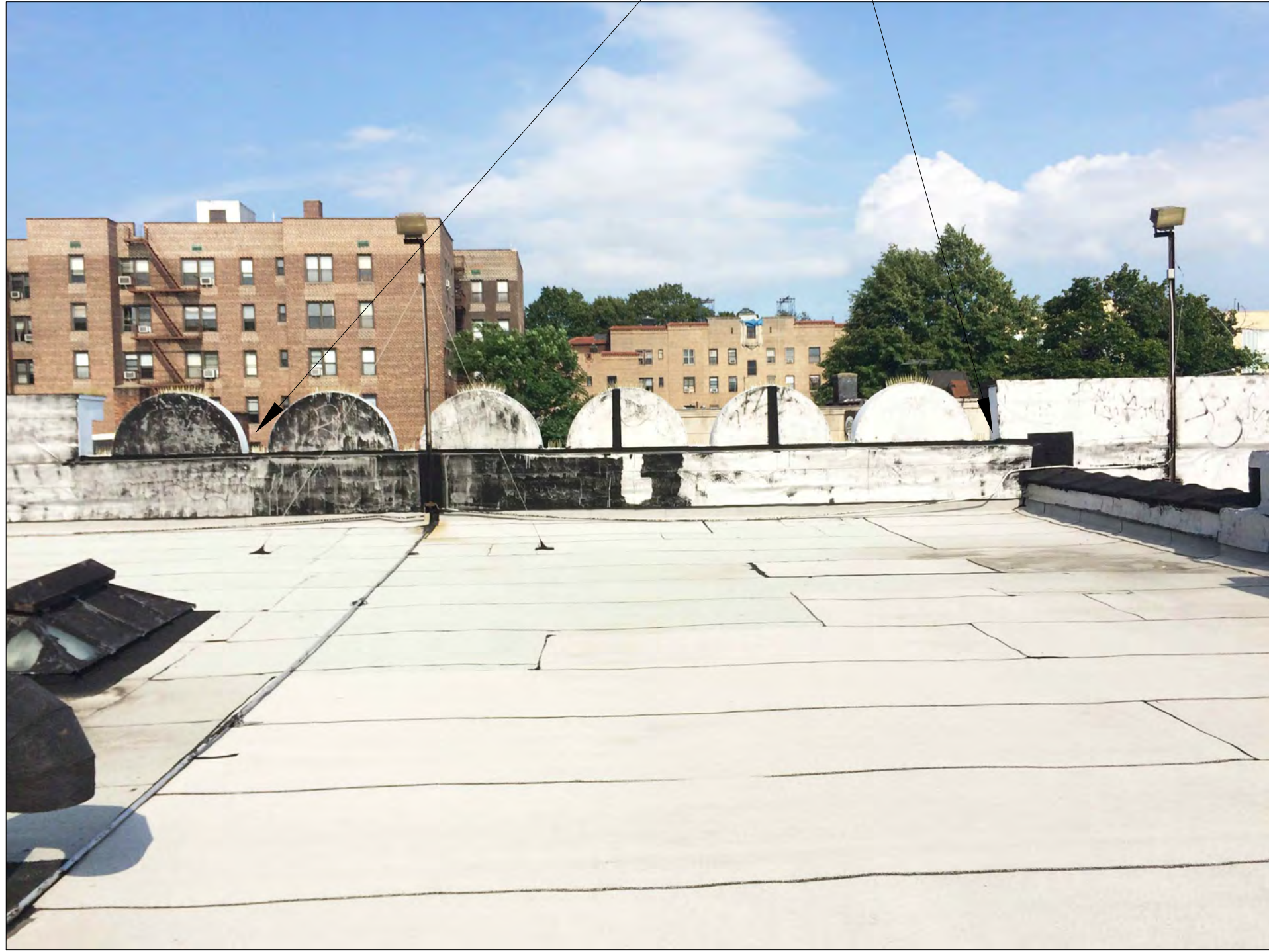
3: ORIGINAL STEPPED PARAPET AND CORNICE HAVE BEEN DEMOLISHED, AS VISIBLE FROM ROOF
