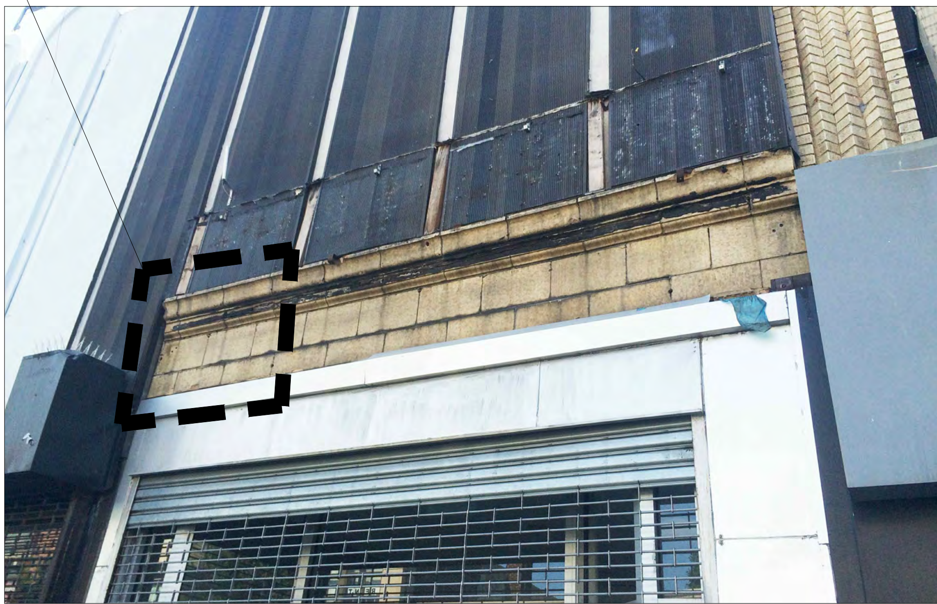
4: REMAINING PORTION OF ORIGINAL LOWER CORNICE LINE AND FACING BELOW ORIGINAL WINDOW SILL
