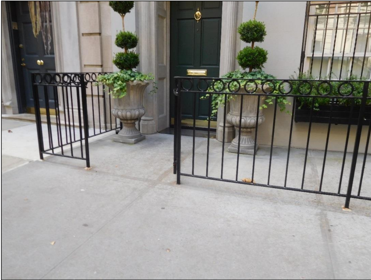
The areaway railing at 126 East 73 rd Street
