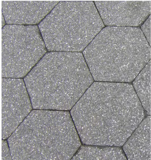
Asphalt Hex Block Pavement
