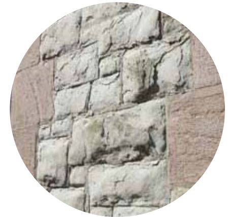
COATING REMOVAL, REPAIR, AND REPOINTING OF SANDSTONE
