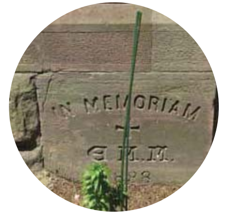
REPAIR BROWNSTONE CRACK WITH COMPOSITE MORTAR
