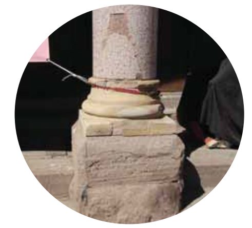
SANDSTONE AND GRANITE PATCH REPAIR
