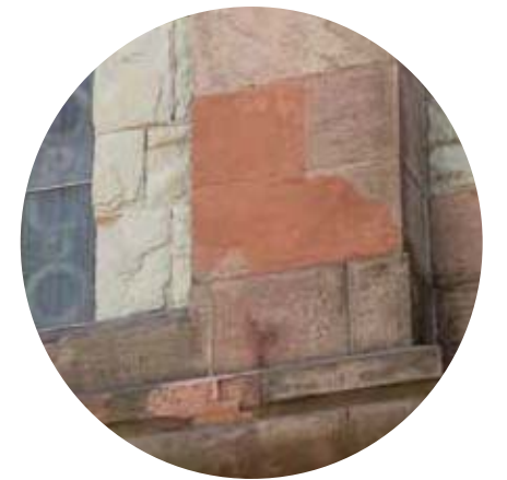
BROWNSTONE INCOMPATIBLE PATCH REMOVAL AND REPLACEMENT
