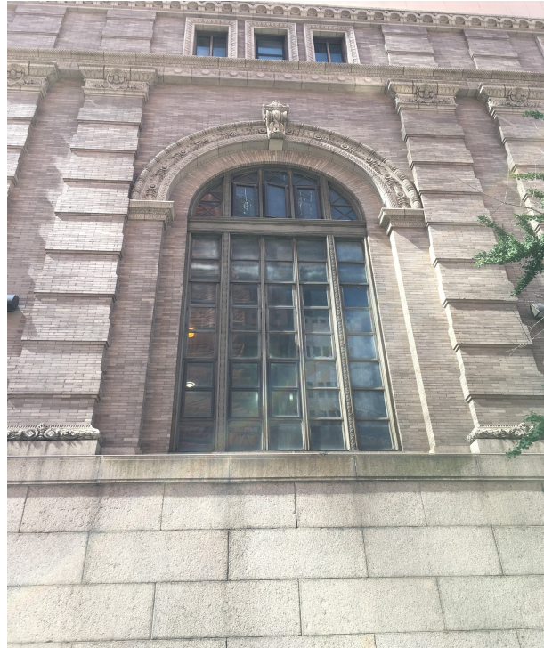
Glazed upper panel, all grillwork in missing 9 Bays
