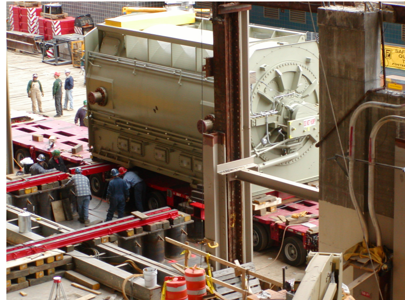
Generator being installed at East River Generating Station
