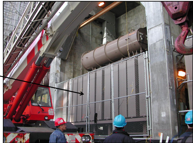
Example of transformer in interior vault
