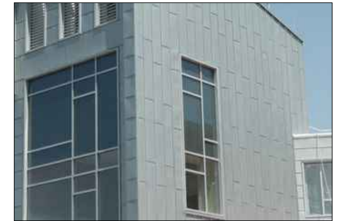
1a FLAT SEAM TERNE EXAMPLE SCALE: 1/2" = 1'-0"
