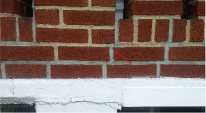
Photo 9: Porch Barrier Crack (Detail)
