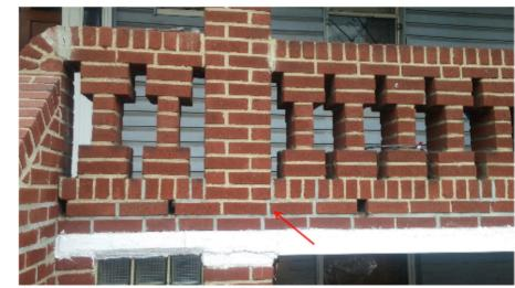
Photo 8: Porch Barrier Crack
