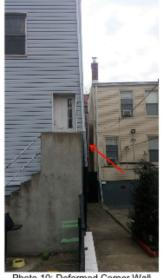
Photo 10: Deformed Corner Wall
