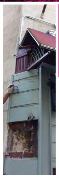
"...there is no evidence of any limestone behind the facade panels. The limestone begins above the graphic signage."
