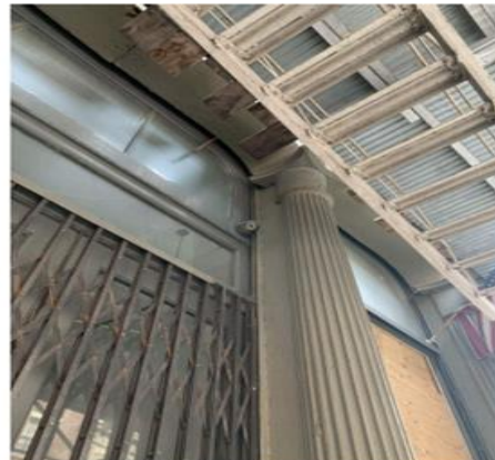
EXISTING CAST IRON ROUND COLUMN CONDITION 2
