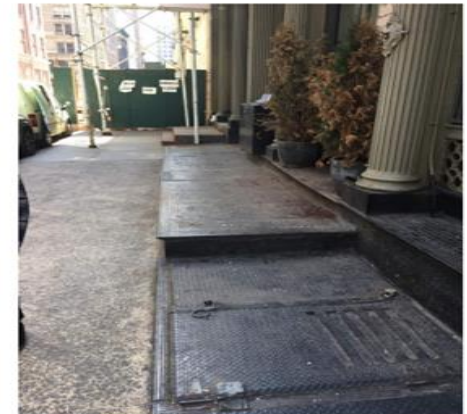
EXISTING SIDEWALK VAULT DOOR
