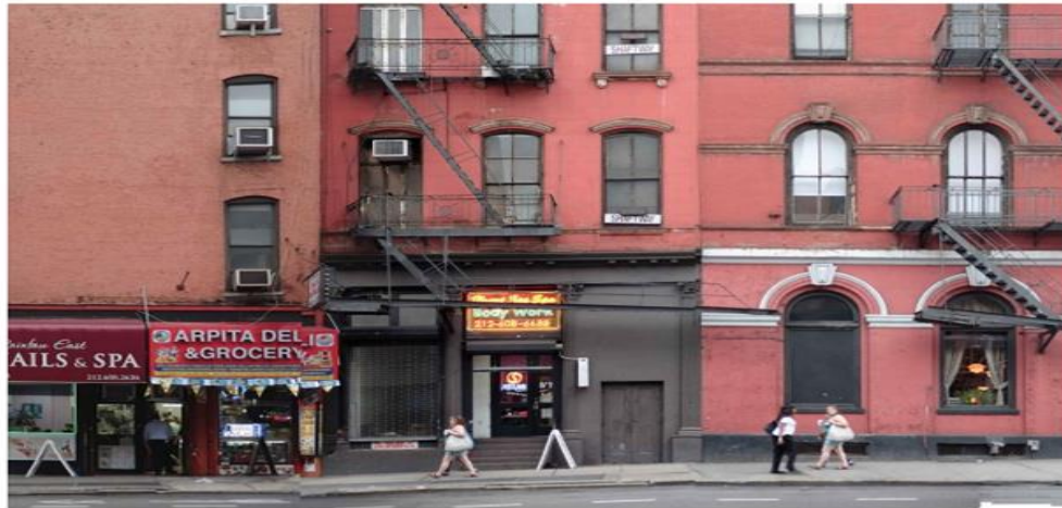
01 VIEW OF EXISTING STOREFRONT – ELEVATION NTS
