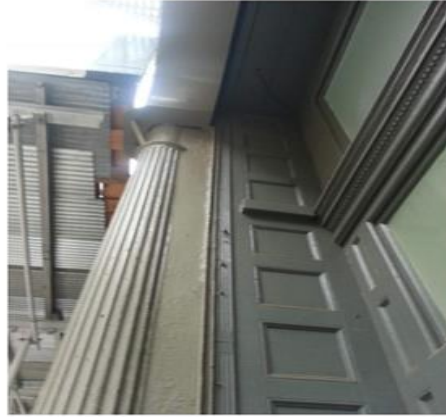
EXISTING CAST IRON ROUND COLUMN CONDITION 1
