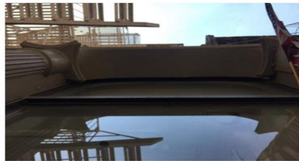
EXISTING STOREFRONT WINDOW CONDITION
