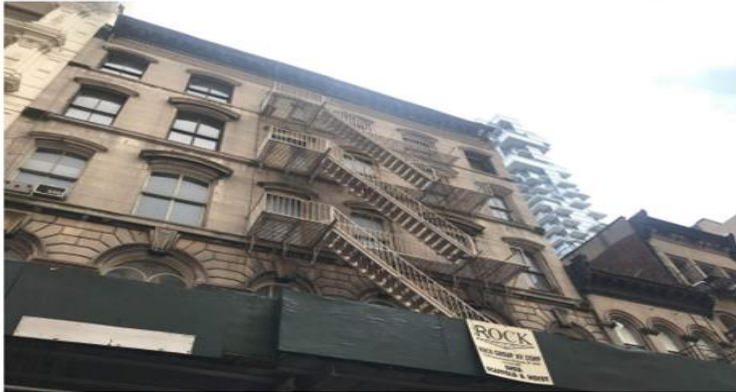
EXTERIOR CLOSE-UP PHOTO (2021)
