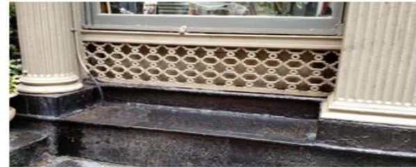
EXISTING CAST IRON GRILLE
