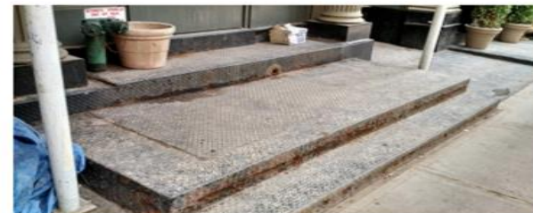
EXISTING DIAMOND PLATE VAULT COVER
