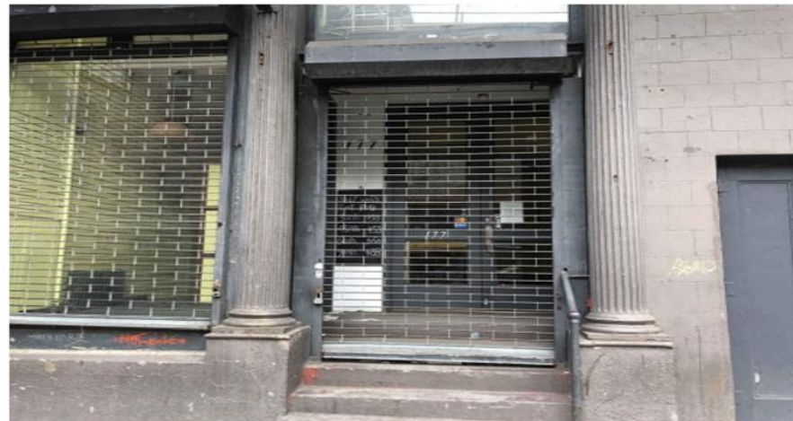
04 PHOTO OF EXISTING RETAIL ENTRY BAY @ STOREFRONT N.T.S.
