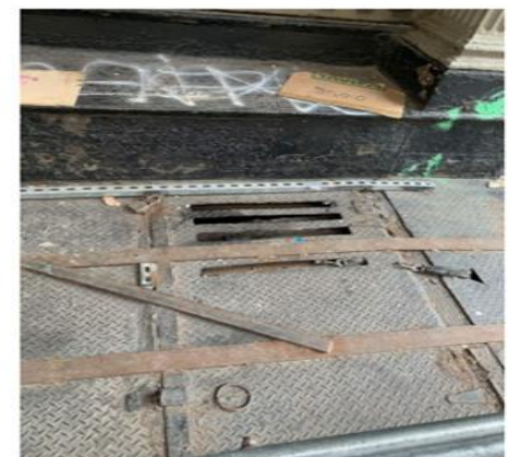
EXISTING SIDEWALK VAULT DOOR
