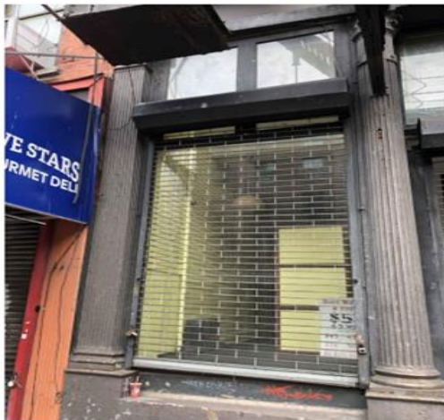
05 PHOTO OF EXISTING RETAIL WINDOW BAY @ STOREFRONT N.T.S.
