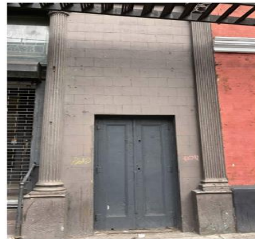
03 PHOTO OF EXISTING ELEVATOR BAY @ STOREFRONT N.T.S.
