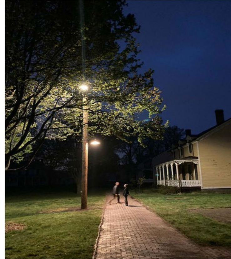
Left: Photograph of lighting mock-up in Nolan Park with Building 9 at background. Right: Photograph of same mock-up showing the combination moonlight and streetlight on one post.
