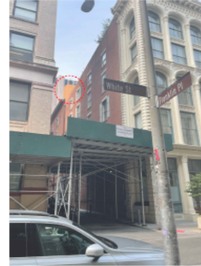
D8 White Street - SE View Proposed Roof Structure - Mock-up
