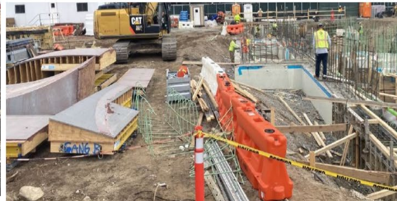
Foundation Work – Wagner Park Pavilion
