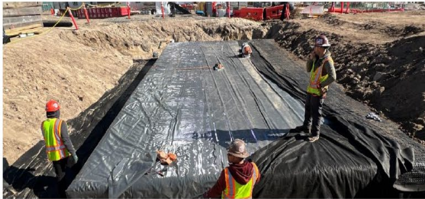
Cistern Installation – Wagner Park
