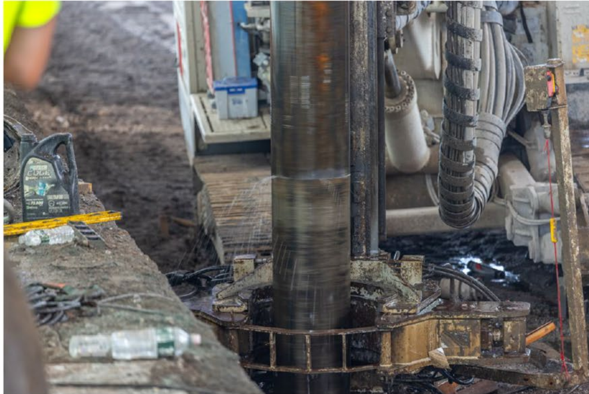
Micropile Installation - September 2023
