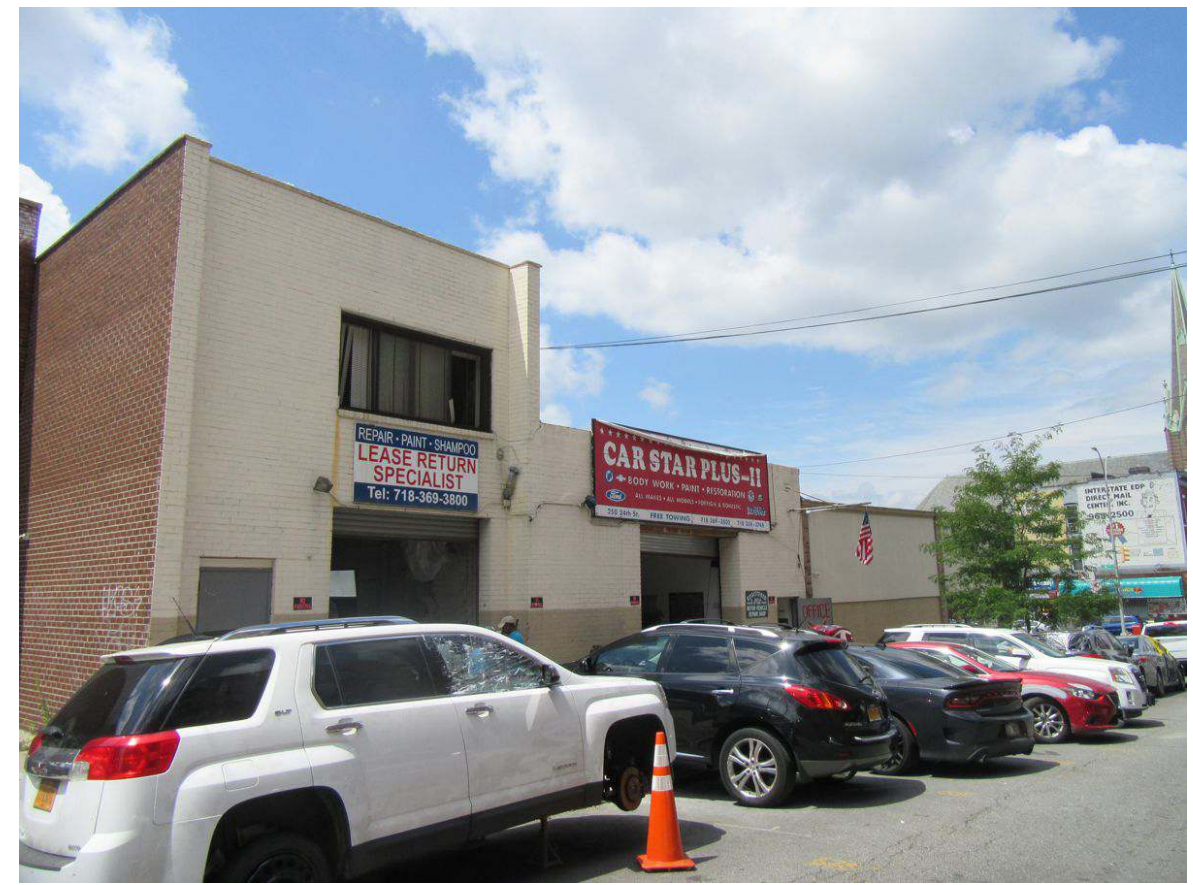
14. View of the Project Area facing west from 24th Street.
