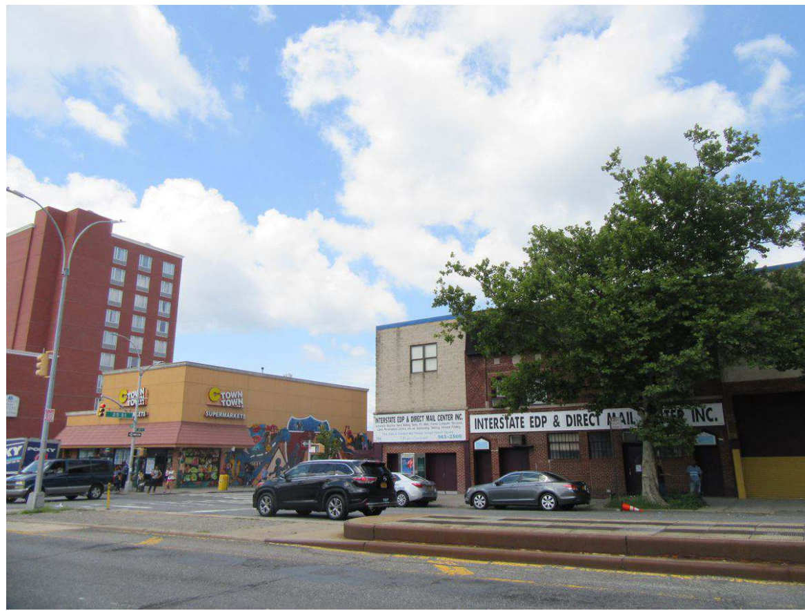
22. View of the northwest side of 4th Avenue facing west from the Development Site.
