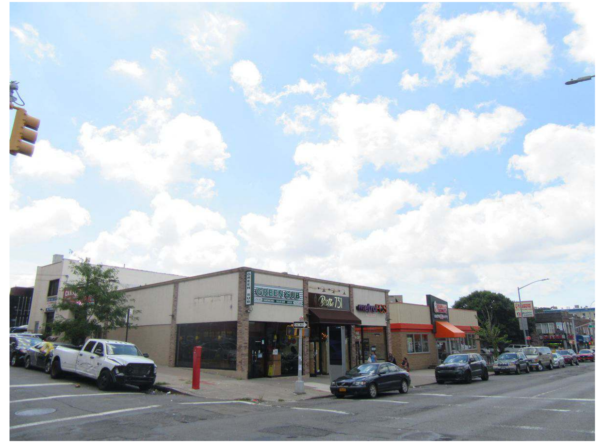
11. View of the Project Area facing south from the intersection of 4th Avenue and 24th Street.
