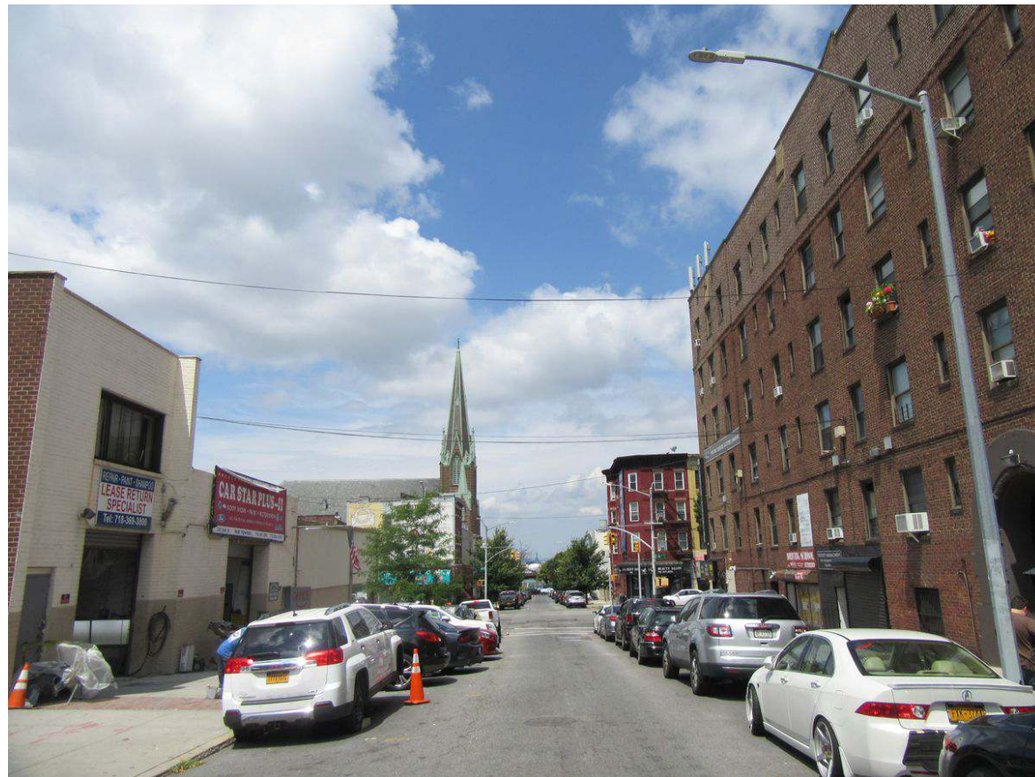
15. View of 24th Street facing northwest (Project Area at left).
