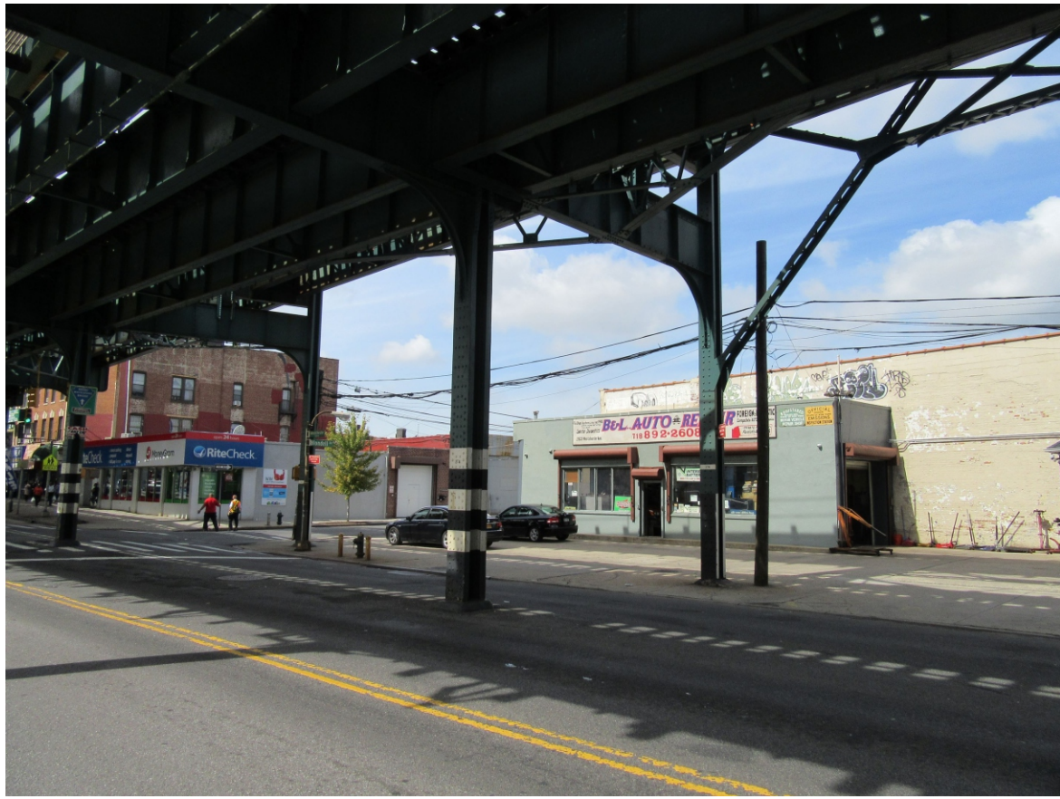
28. View of the north side of Westchester Avenue facing northwest toward Blondell Avenue.
