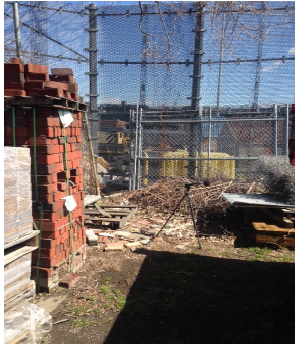
Photo 4: Noise Monitoring Location Four (4) at the Frontage of Westchester Ave.
