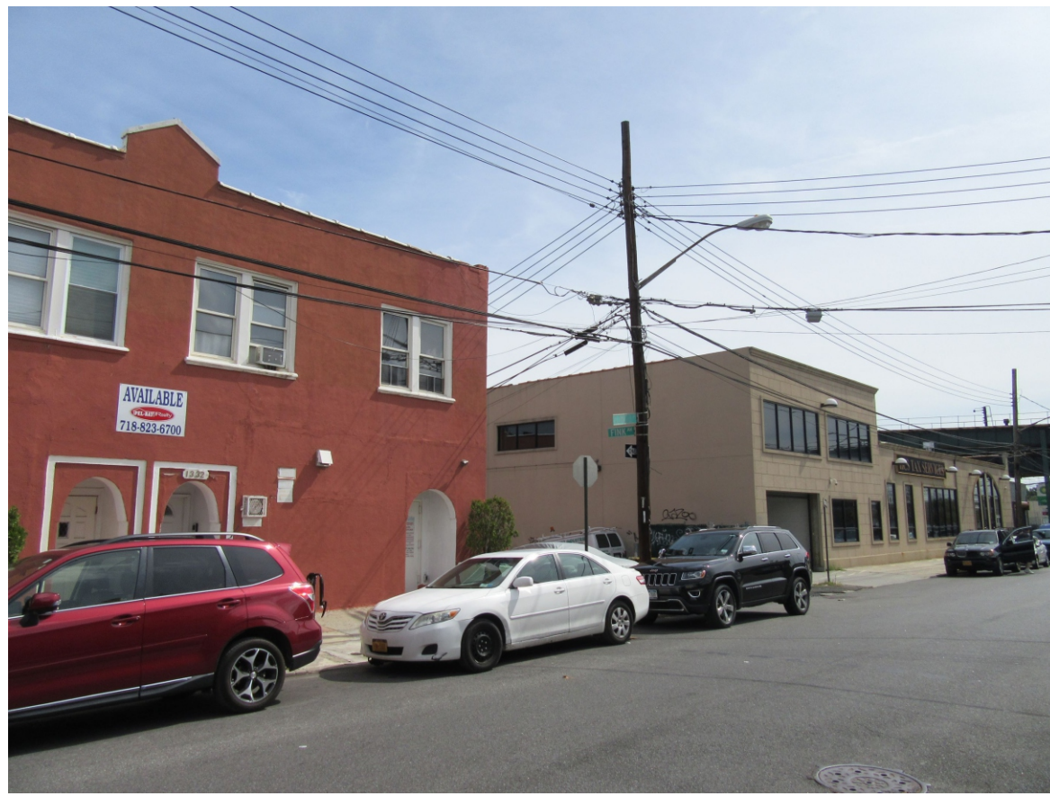
10. View of the east side of Blondell Avenue facing southeast toward Fink Avenue.
