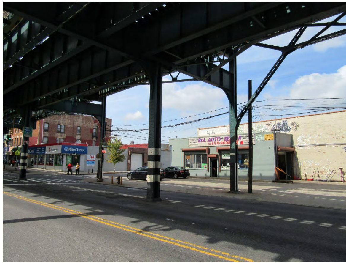
28. View of the north side of Westchester Avenue facing northwest toward Blondell Avenue.
