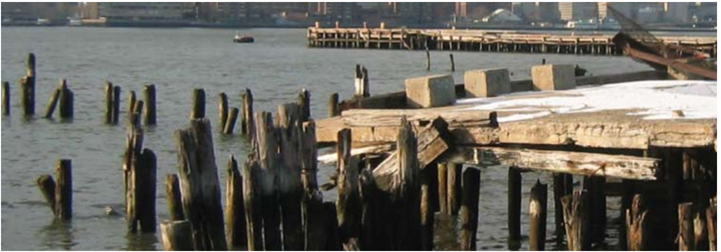
Without regular maintenance, piers will deteriorate until they collapse, as seen with this pier in Greenpoint, Brooklyn. It is difficult to obtain a permit to rebuild.
