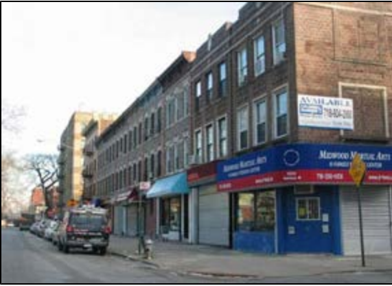
Proposed R5D district at the corner of Avenue H and East 13th Street
