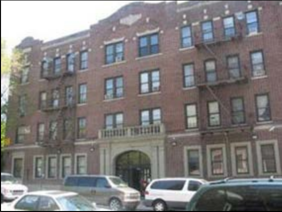
Proposed R6A district along Stratford Road between Caton Avenue and Church Avenue
