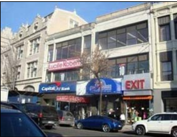
Proposed C4-4A district along Flatbush Avenue, between Church Avenue and Snyder Avenue
