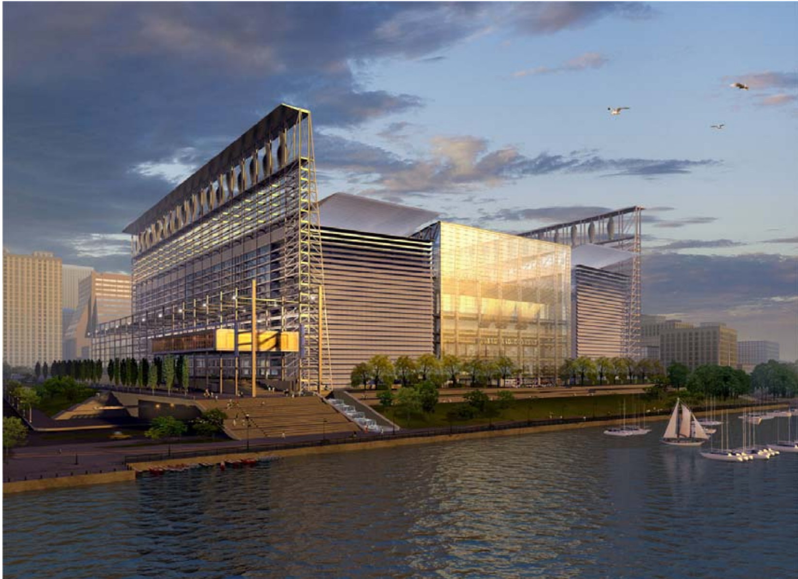
Alternative Q: Proposed Action with Development of a Deck Over Route 9A between the Multi-Use Facility & Hudson River Park, 2025 Build Scenario
