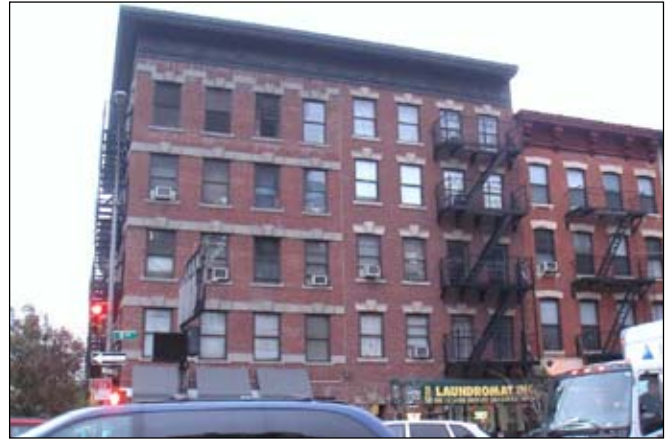
Site 51: Ninth Avenue between West 39th and West 40th Streets
