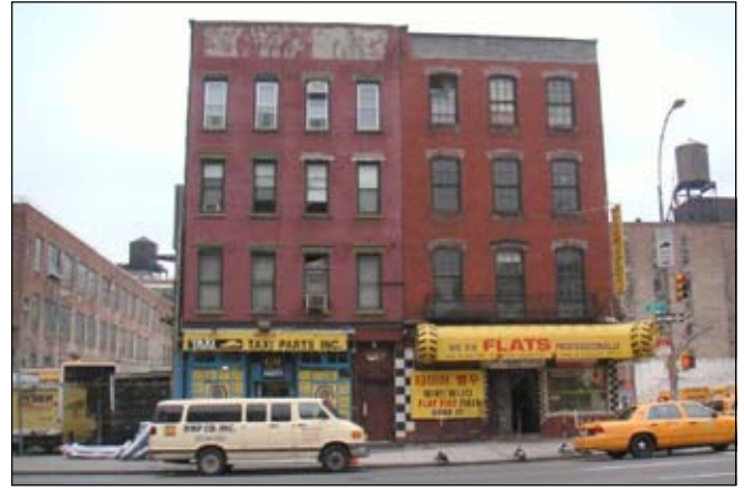
Site 5: Ninth Avenue between West 34th and West 35th Streets
