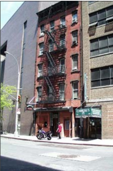
Site 35: West 41st Street between Eighth and Ninth Avenues
