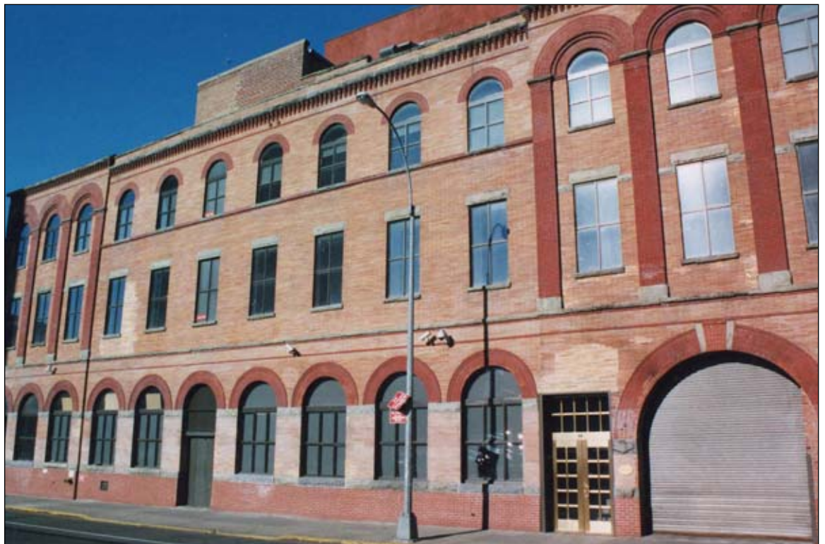
Former Franco-American Baking Company, 509-517 West 38th Street. View north 92
