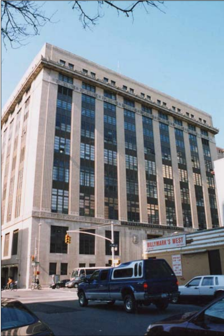
Morgan General Mail Facility. Ninth Avenue facade, view west 17
