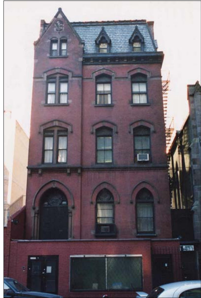
St. John the Baptist Roman Catholic Church, 207-215 West 30th Street. View north 6b
