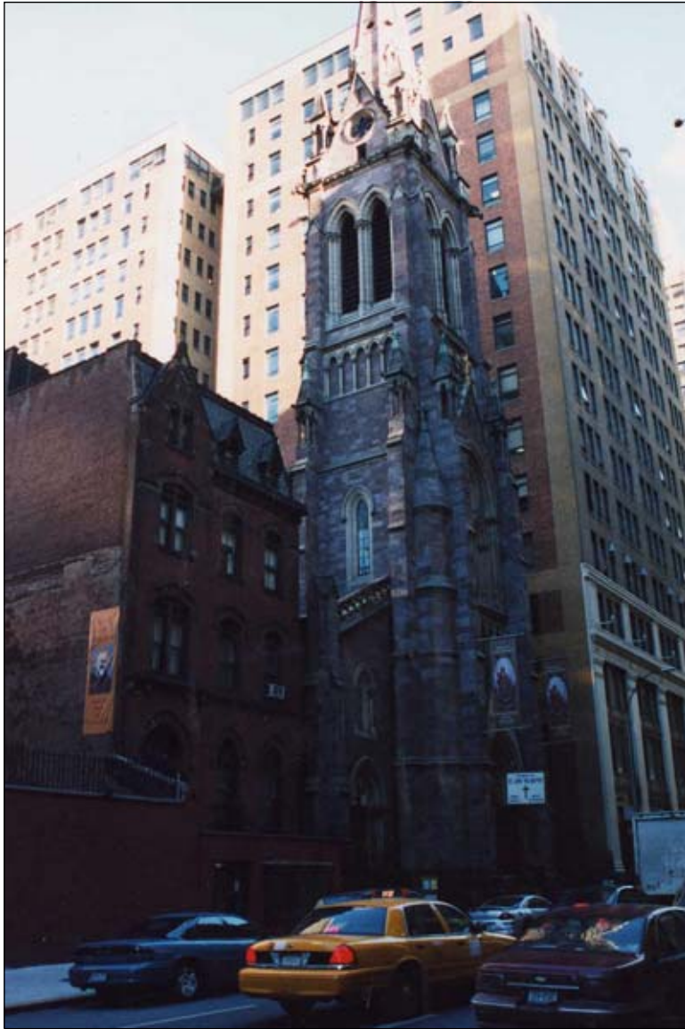
St. John the Baptist Roman Catholic Church, 207-215 West 30th Street. View northeast 6a
