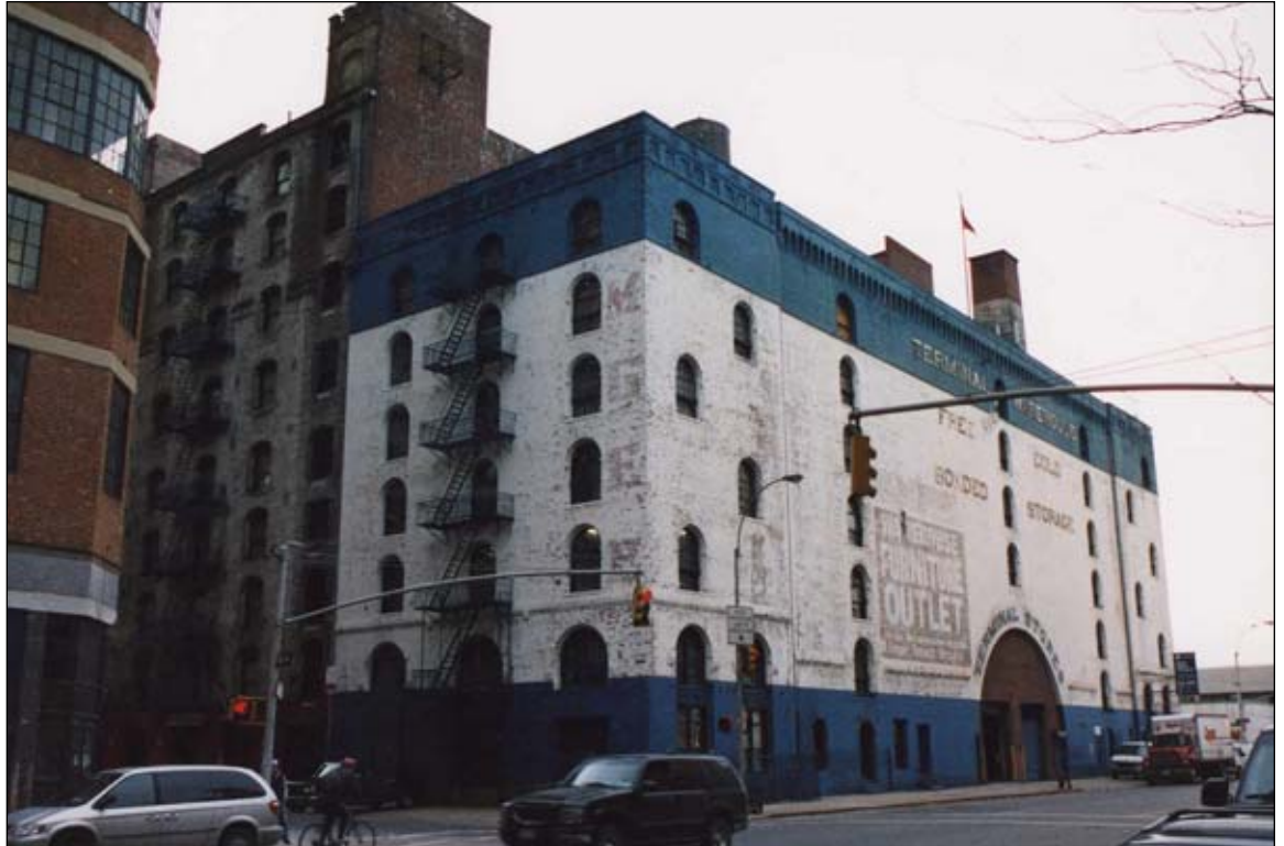
New York Terminal Warehouse Company. Eleventh Avenue facade, view north 23a
