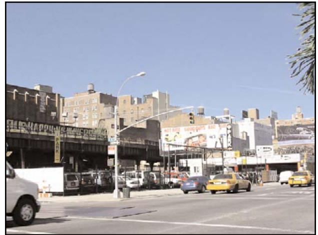
A view facing northwest along the west side of Tenth Avenue from W. 18th Street.
