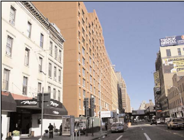
A view facing east along the north side of W. 23rd Street, from Eleventh Avenue.
