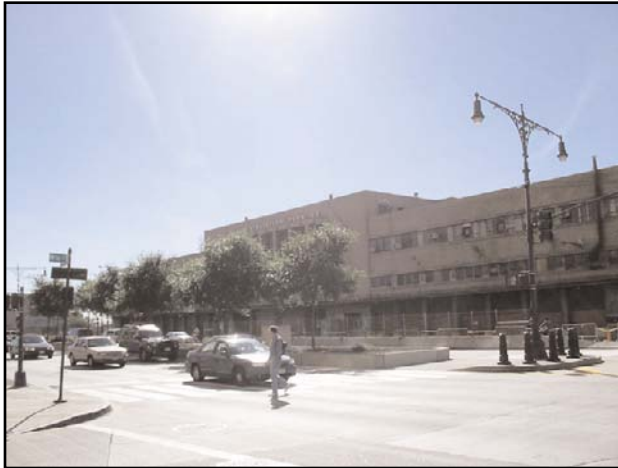
A view of Pier 57 facing southwest from the intersection of W. 13th Street and Route 9A.
