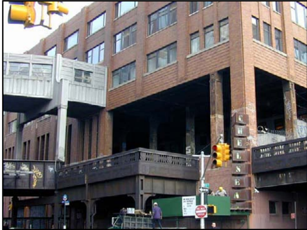
The High Line penetrates the Chelsea Market building underneath an elevated pedestrian connection, (northeast view, Tenth Avenue at W. 15th Street)
