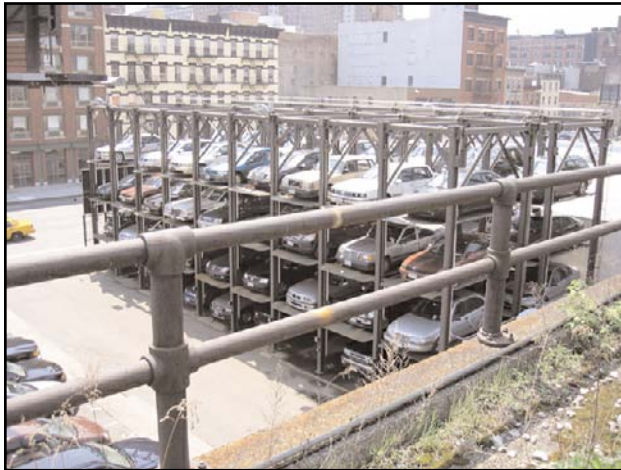
A view facing southeast at parking stackers at Tenth Avenue and W. 21st Street.*
