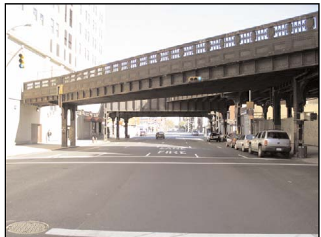
A view facing north along Tenth Avenue from its intersection with W. 16th Street.
