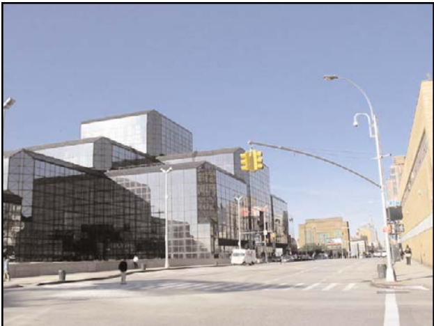
A view facing north along Eleventh Avenue at the Jacob Javitz Convention Center.
