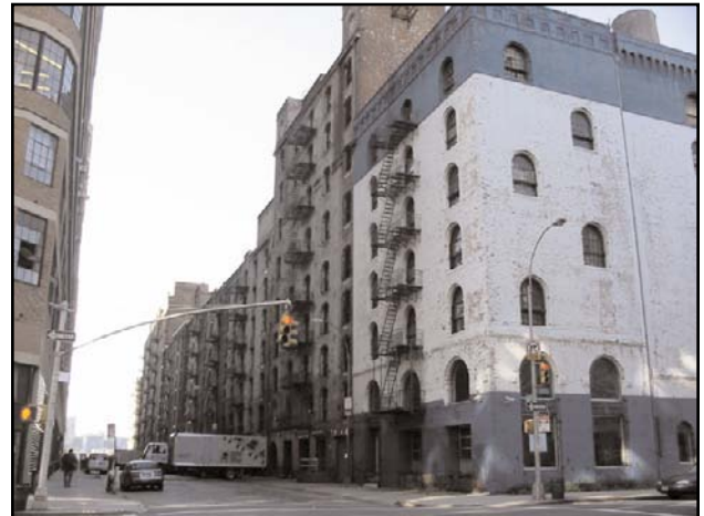
A view of the northwest corner of the intersection of W. 27th Street and Eleventh Avenue.
