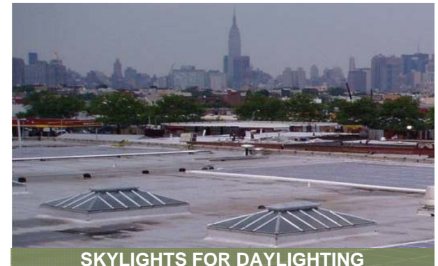
SKYLIGHTS FOR DAYLIGHTING
