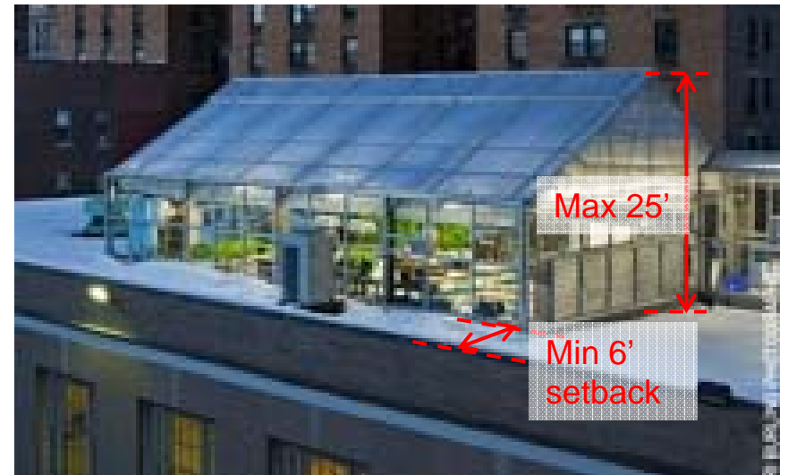
PS 333. Photo by Ari Burling. Courtesy: New York Sunworks.
