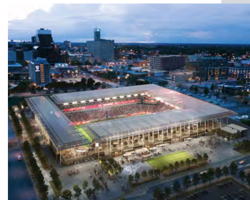
The proposed new MLS stadium in St. Louis, Missouri, invites the surrounding community to experience the spaces surrounding the venue. Image courtesy of HOK/Snow Kreilich Architects.
