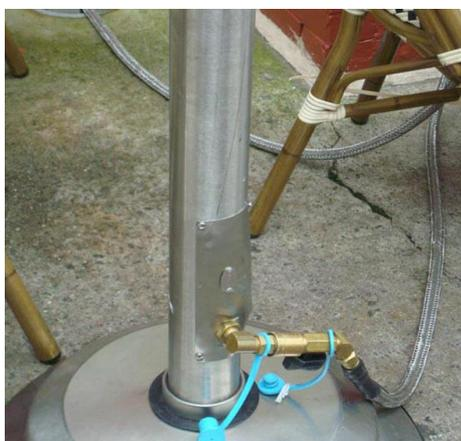
*Flexible gas hose connector at portable gas heater (seen without protective cover)*
