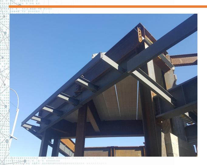
On February 16, a steel worker was installing a beam for the third-floor deck at 556 Bergen Avenue in the Bronx. He slipped off the beam and was stopped from falling by his harness. He sustained some non-life-threatening injuries as he hit a beam during the fall.
