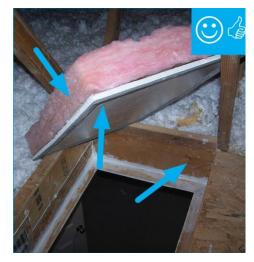
Figure BE-12.b. Access Hatch Properly Insulated Source: basc.pnnl.gov/images
