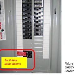
Figure OR-6. Electrical service panel with dedicated breaker for future PV system Source: basc.pnnl.gov/images
