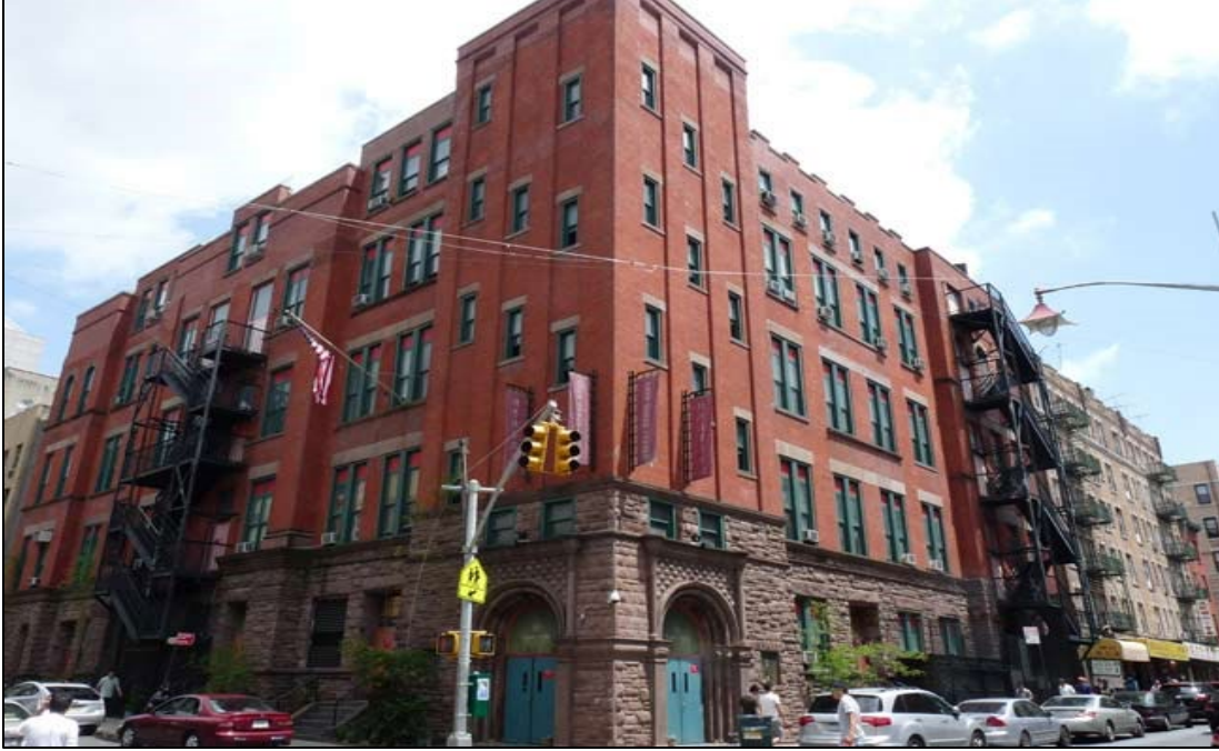
Figure 1: 70 Mulberry Street prior to fire.
