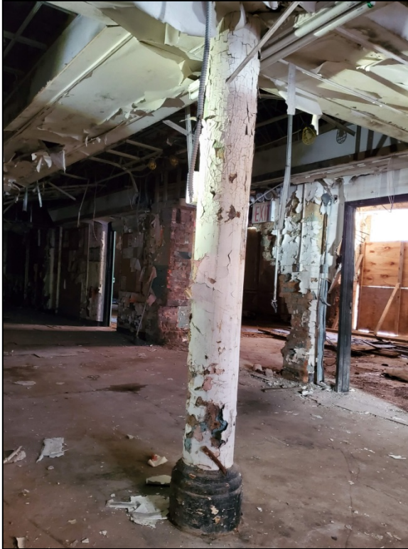
Figure 37: Cast Iron columns.
