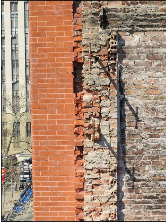
Figure 25: Demolition on corner of stair tower, Bayard Street.
