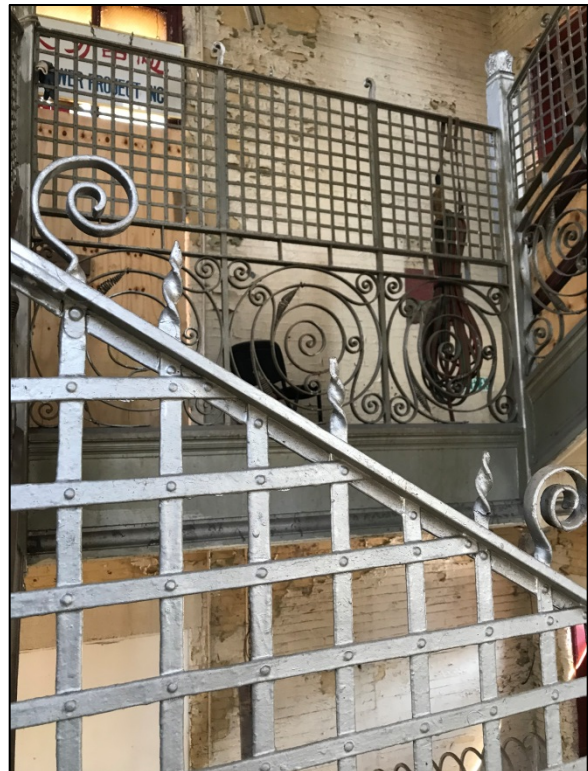
Figure 48: Wrought iron railing.
