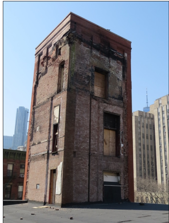
Figure 24: Interior exposed walls of stair tower.
