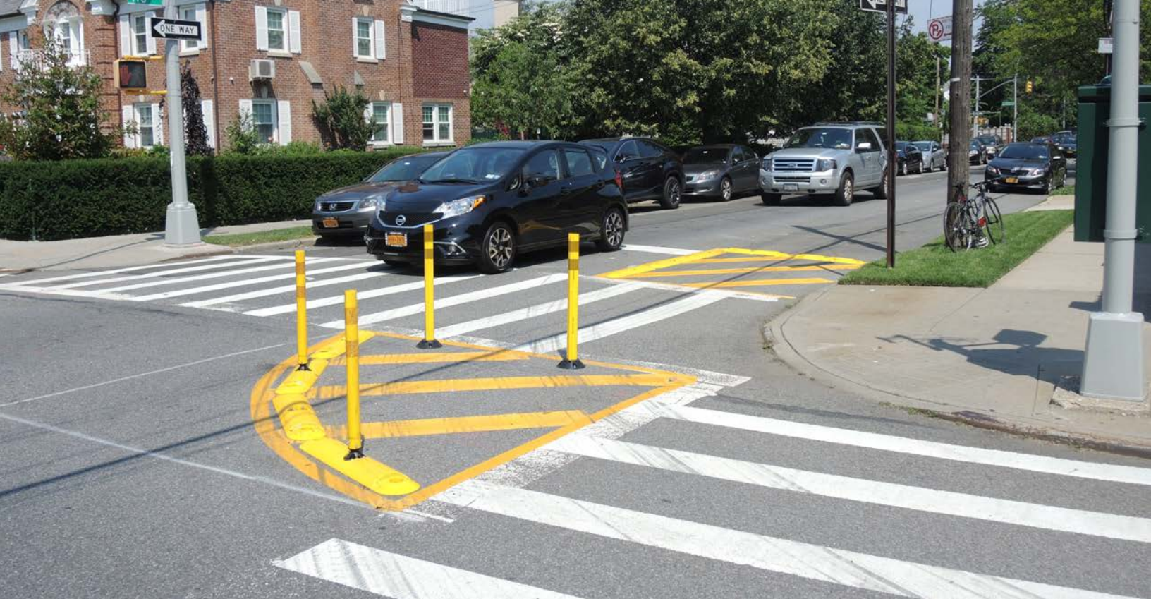
Above: slow turn wedge - markings and plastic delineators within the intersection.
