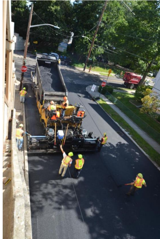
NYC DOT testing soy-bio based asphalt on NYC Street.
