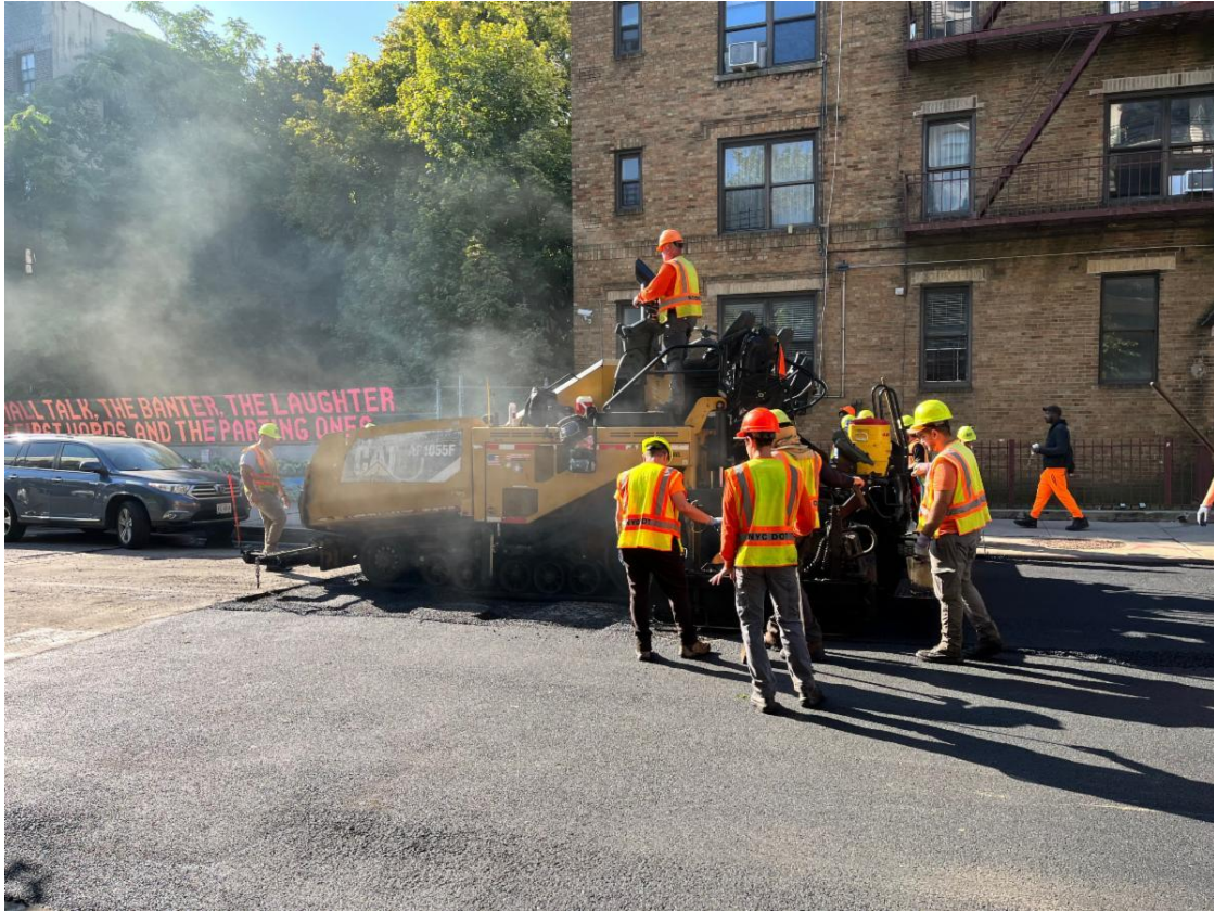
NYC DOT Paving Crew in Brooklyn, New York.
