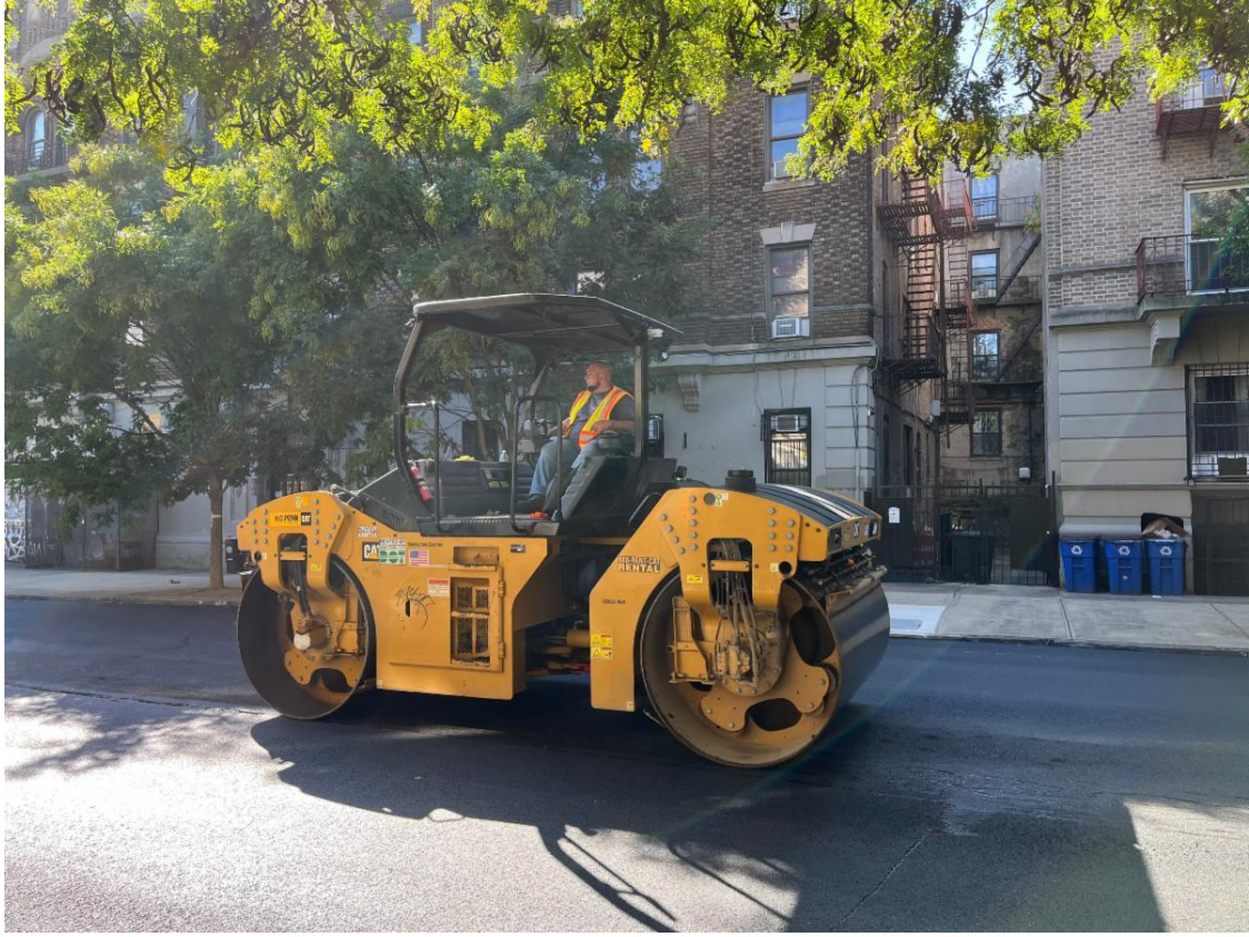
NYC DOT Roller used to compact asphalt on NYC street.
