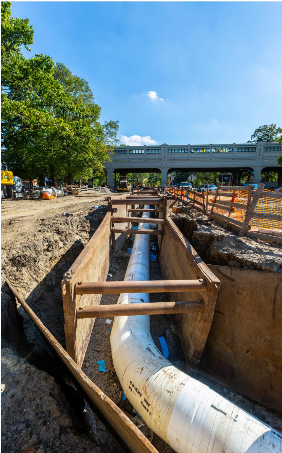
**WATER MAINS** are pipes that deliver water. New York City has thousands of miles of underground water mains. These pipes bring water into homes, schools, hospitals, and businesses throughout the five boroughs. Some of these pipes are over 100 years old and they need to be replaced as they age. The New York City Department of Design and Construction (DDC) installs new or replaces old pipes to deliver high-quality water for decades to come.
