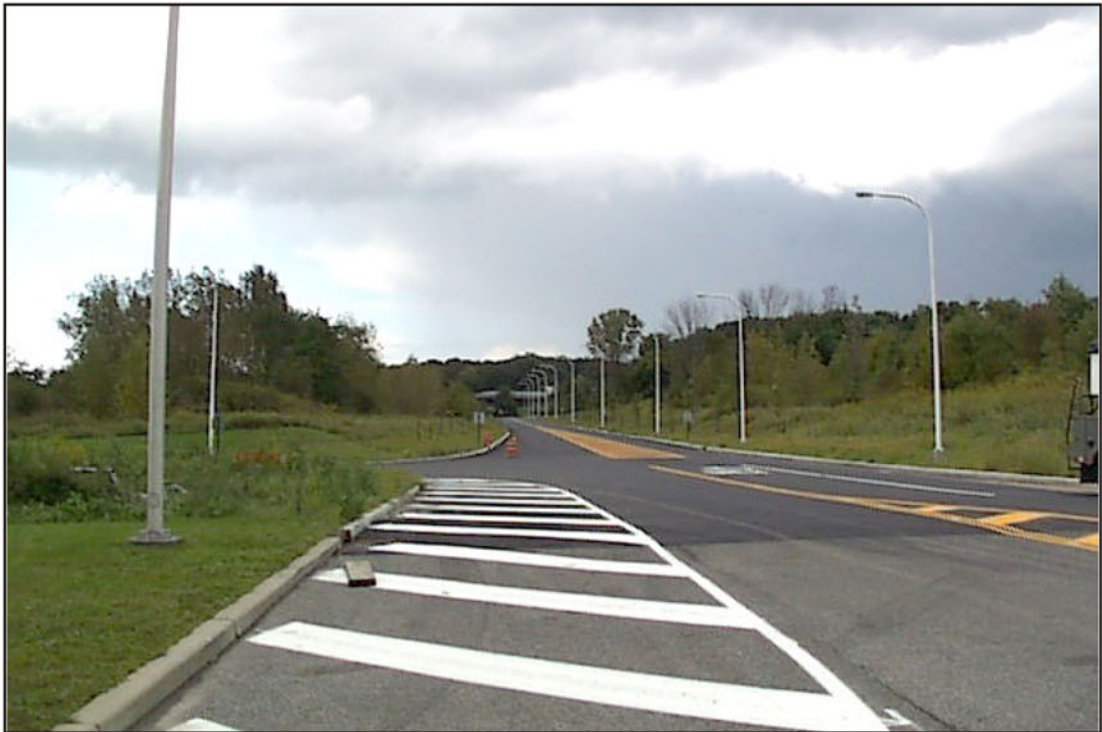
Photograph 4 - View north on Walker Road. Western edge of Eastview Site.
