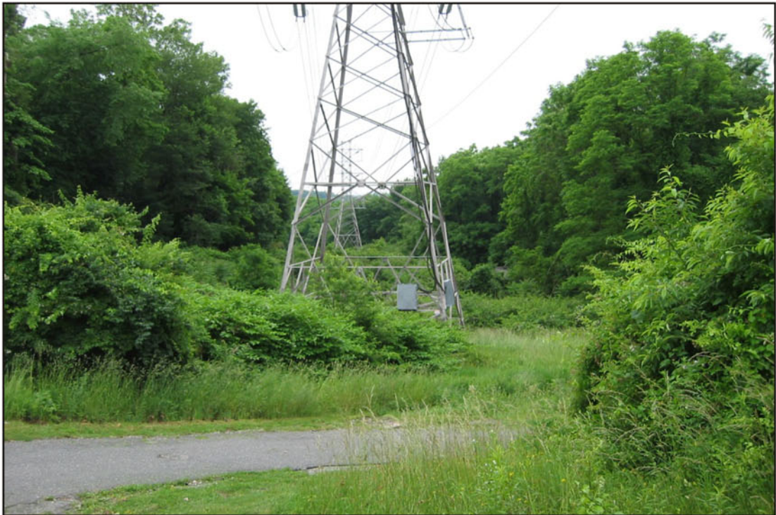
Photograph 6 - View south of transmission lines near Grasslands Road near Catskill Connection Chamber.
