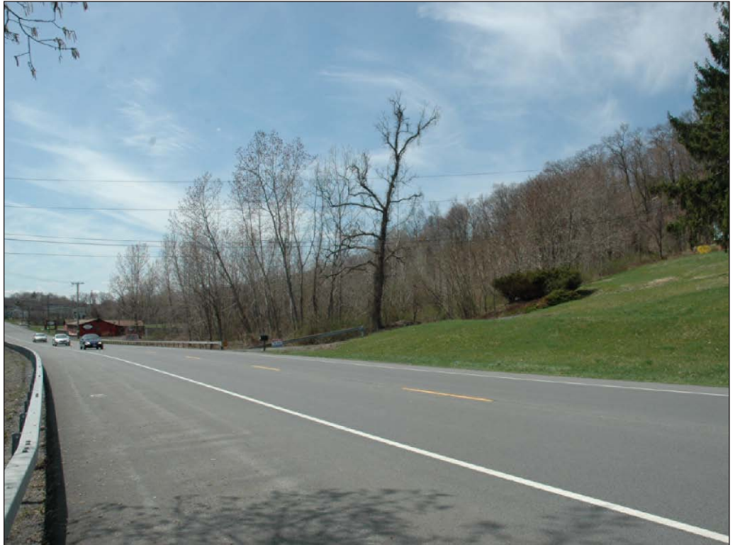
View looking southwest toward West Connection Site from Route 9W 3
