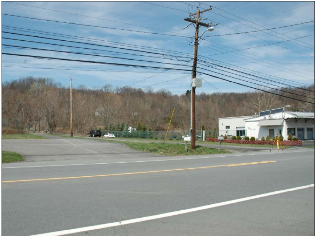
View of West Connection Site (looking northwest) 2
