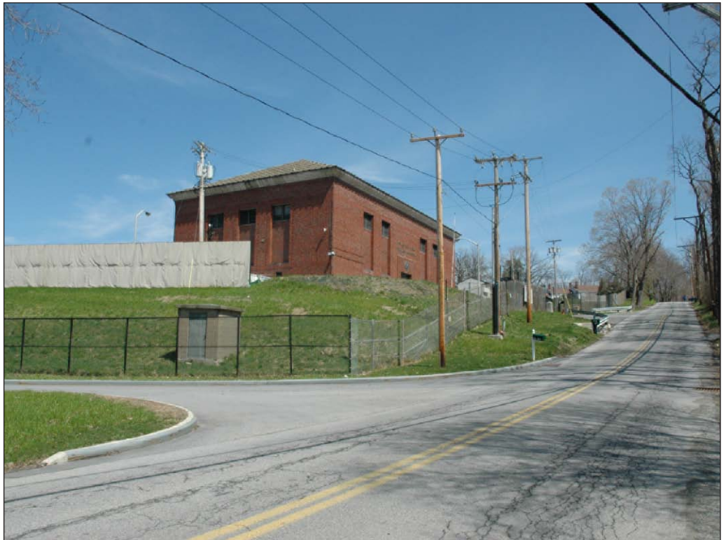
View of East Connection Site (looking northwest) 5
