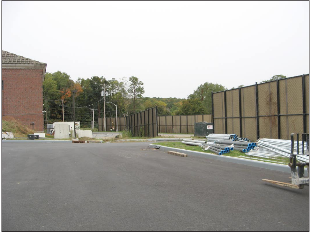
Shaft building from trailer parking lot facing east 5
