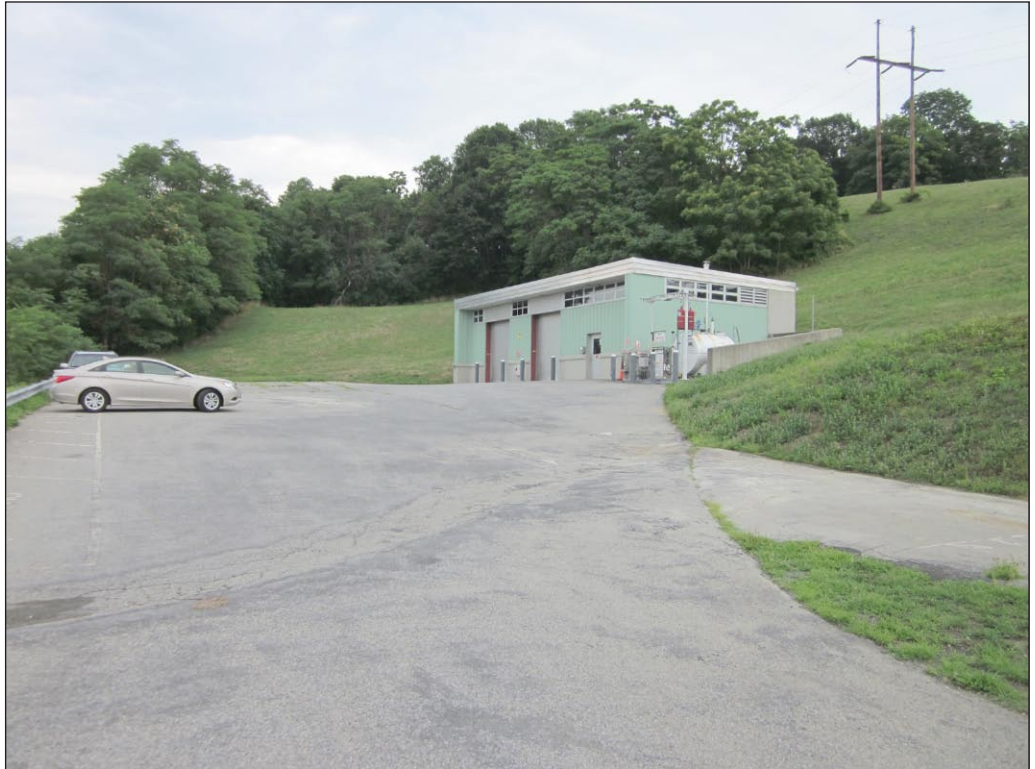
Northwest building from southern access road facing north-northeast 3
