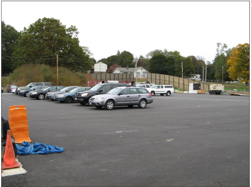
Trailer parking lot facing northeast 6
