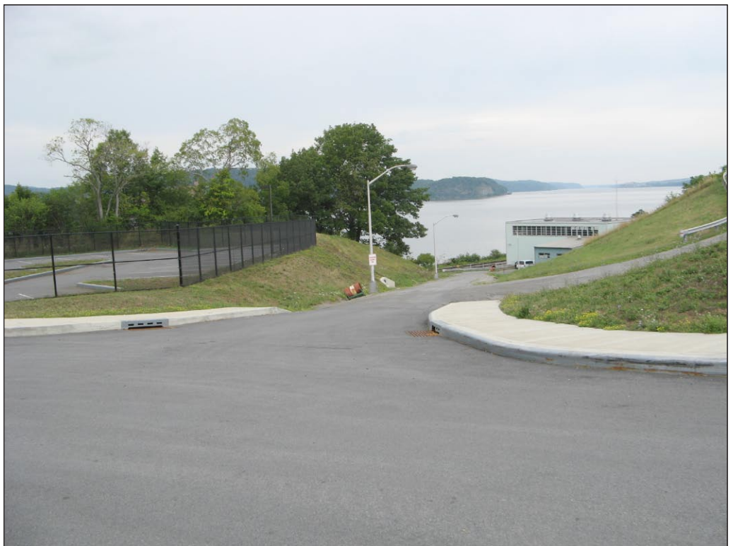
Southwest building from main entrance facing west 2
