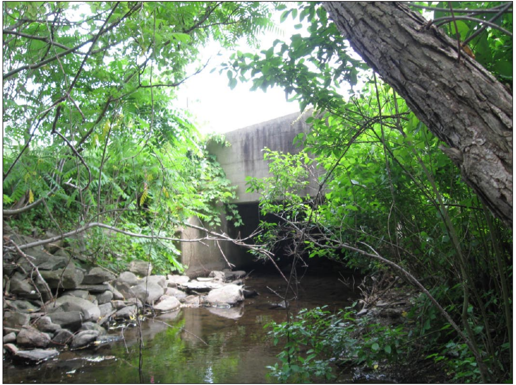
Culvert under 9W 6.10.11 1
