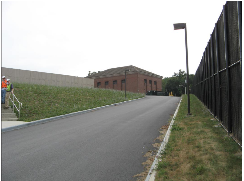
Shaft building from main entrance facing east 1
