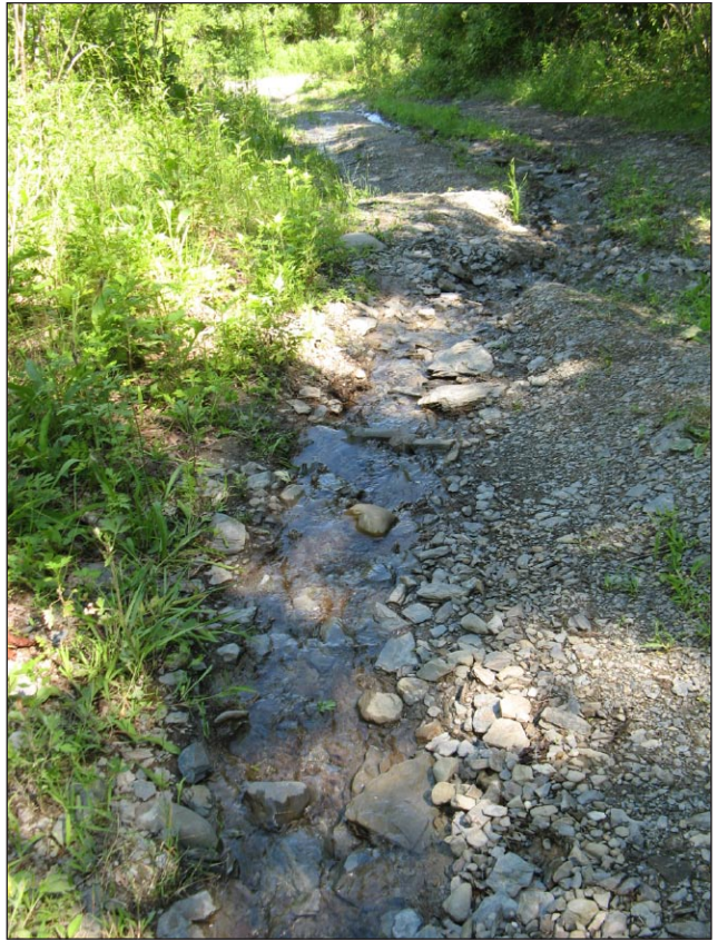
Water flowing from spring in dirt access facing down slope 6.29.11 9
