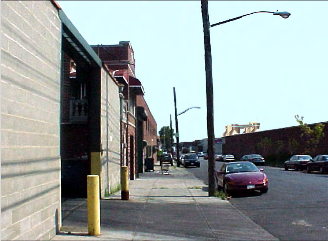
Illustrative Rendering: View south on Coster Street from Oak Point Avenue E
