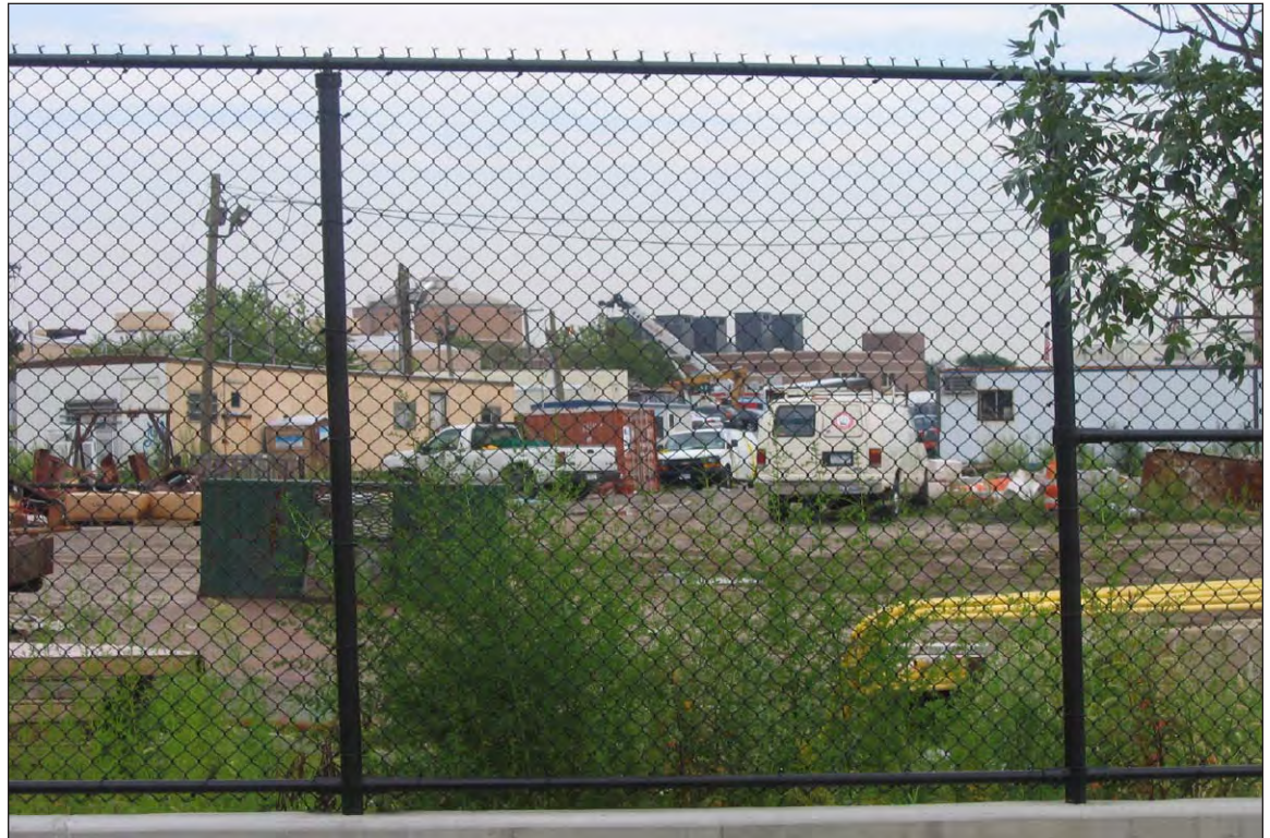
View of the construction staging area from Barretto Point Park 6
