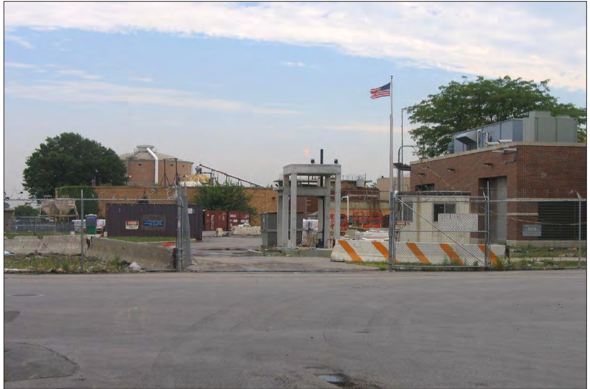
Project site entrance at Ryawa Avenue and Coster Street 3
