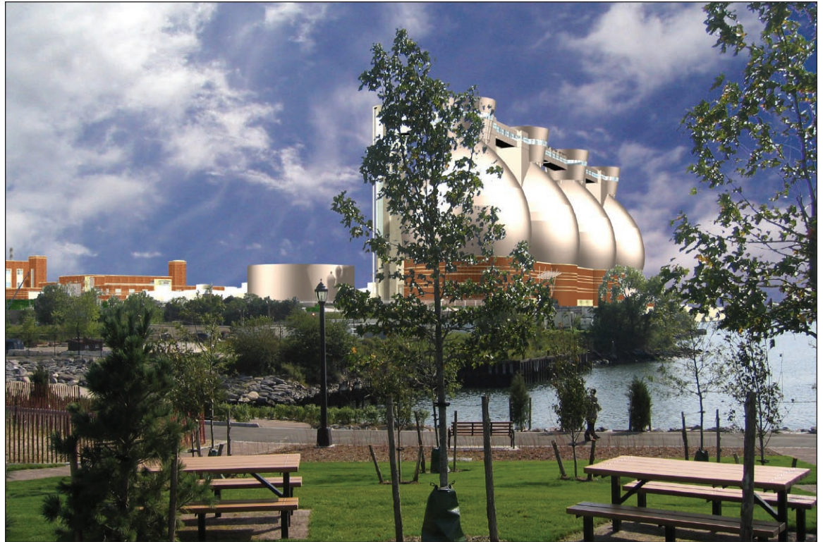
View southeast from within existing Barretto Point Park 1
