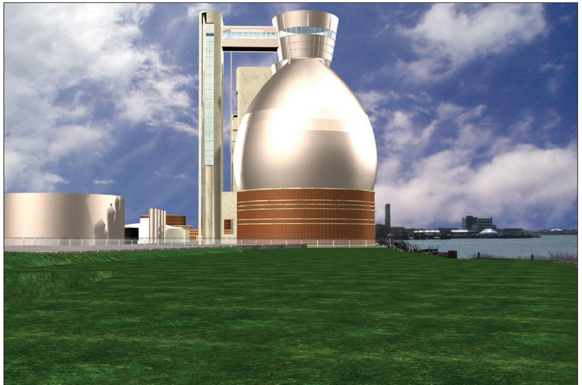
View south from construction staging area (future Barretto Point Park) 2
